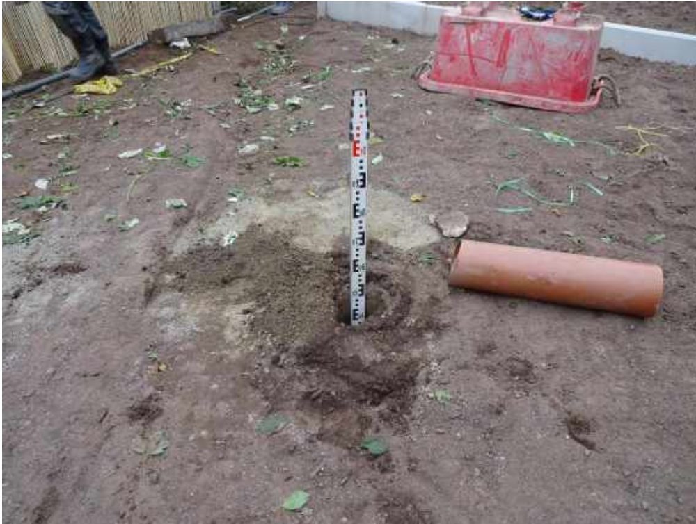
Photograph 11 Plot 19 rear garden with granular subbase visible on the surface.
