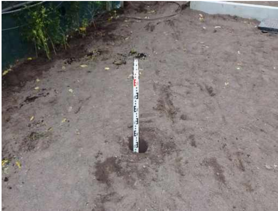
Photograph 5 Rear garden of Plot 8 with 600mm capping.
