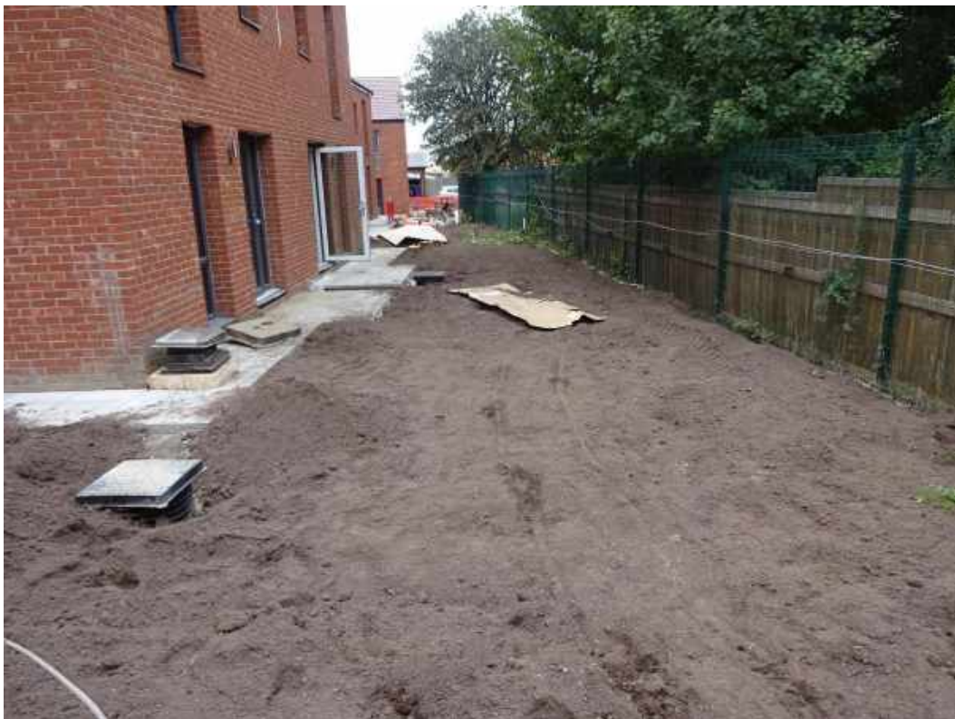
Photograph 1 Compacted subsoil to Plot 3 during installation.
