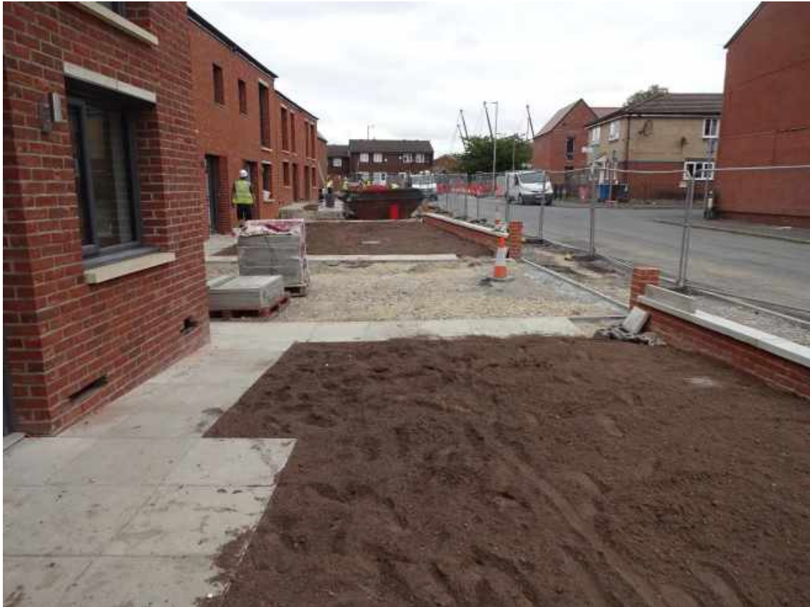
Photograph 13 Plot 10 to 16 front gardens with granular subbase just visible.
