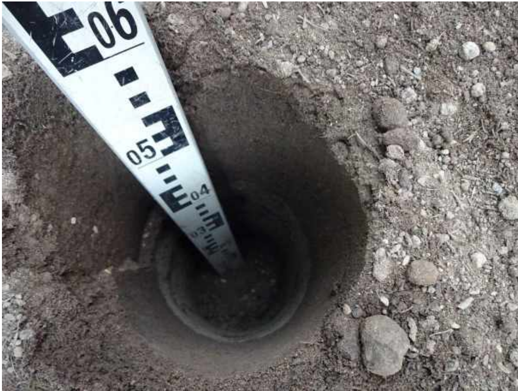
Photograph 7 Plot 8 rear garden with granular subbase just visible.
