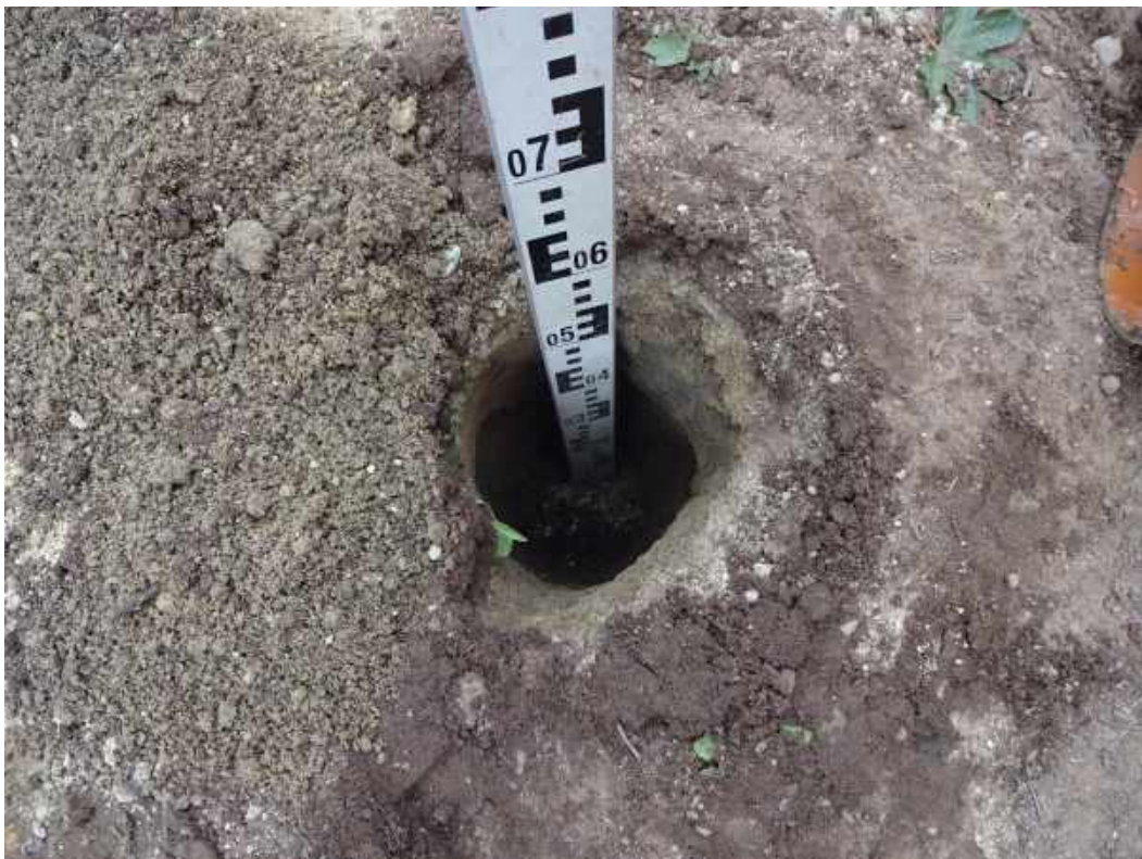
Photograph 12 Plot 19 rear garden with granular subbase visible at 150mm.
