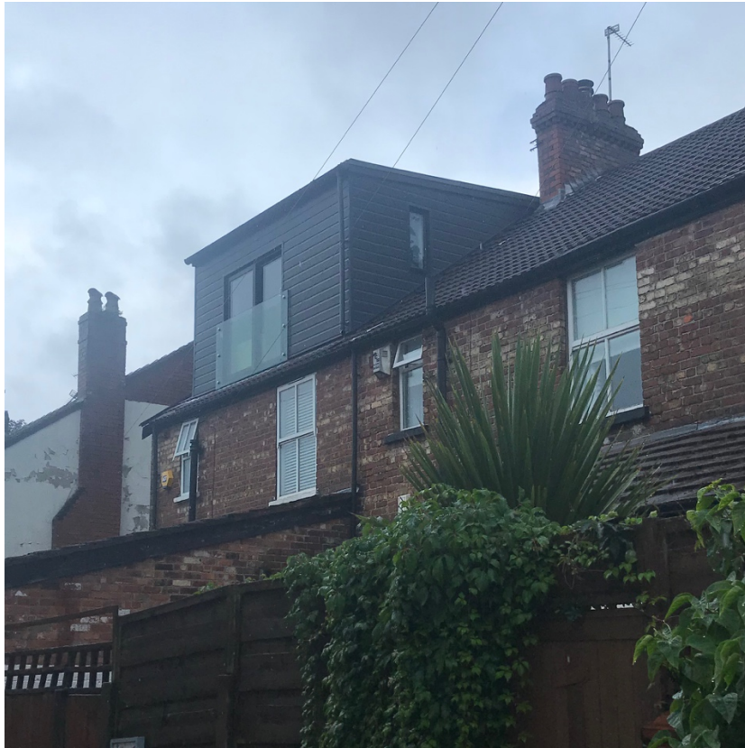
69 Whalley Road Permission no. 113696_FH_2016
