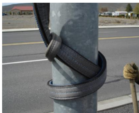
Example of sling attachment
