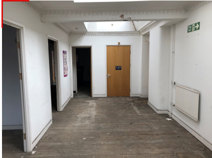
PHOTOGRAPH OF CIRCULATION LOBBIES AND DOORS TO WC'S SHOWING HOW THE EXISTING CEILING JOISTS ABOVE HAVE BEEN UNDERDRAWN WITH MODERN PLASTERBOARD AND SKIM FINISH, PAINTED WITH WHITE EMULSION AND THE SUBSEQUENT INSTALLATION OF MODERN SPOT DOWNLIGHTERS. CORNICE TO CIRCULATION LOBBY IS NON-ORIGINAL.
