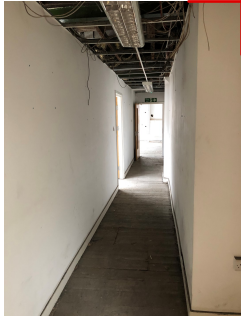
PHOTOGRAPH OF CIRCULATION LOBBIES WITH MODERN SUSPENDED CEILING & MODULAR LIGHTING WITHIN. CEILING TILES HAVE SUBSEQUENTLY BEEN REMOVED TO REVEAL CEILING JOISTS AND TIMBER BEAMS ABOVE
