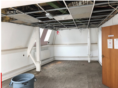
PHOTOGRAPH OF MODERN SUSPENDED CEILING & MODULAR LIGHTING WITHIN. CEILING TILES HAVE SUBSEQUENTLY BEEN REMOVED TO REVEAL CEILING JOISTS AND TIMBER BEAMS ABOVE
