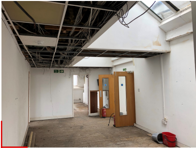
PHOTOGRAPH OF SLOPING CEILING/ROOF ADJACENT TO MODERN RETROFIT SUSPENDED CEILING WITH IN-LINE GEORGIAN WIRED TIMBER WINDOWS
