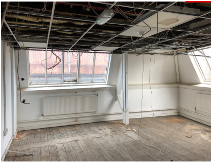
PHOTOGRAPH OF MODERN SUSPENDED CEILING & MODULAR LIGHTING WITHIN. CEILING TILES HAVE SUBSEQUENTLY BEEN REMOVED TO REVEAL CEILING JOISTS AND TIMBER BEAMS ABOVE
