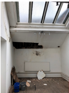
PHOTOGRAPH OF SLOPING CEILING/ROOF WITH IN-LINE GEORGIAN WIRED TIMBER WINDOW
