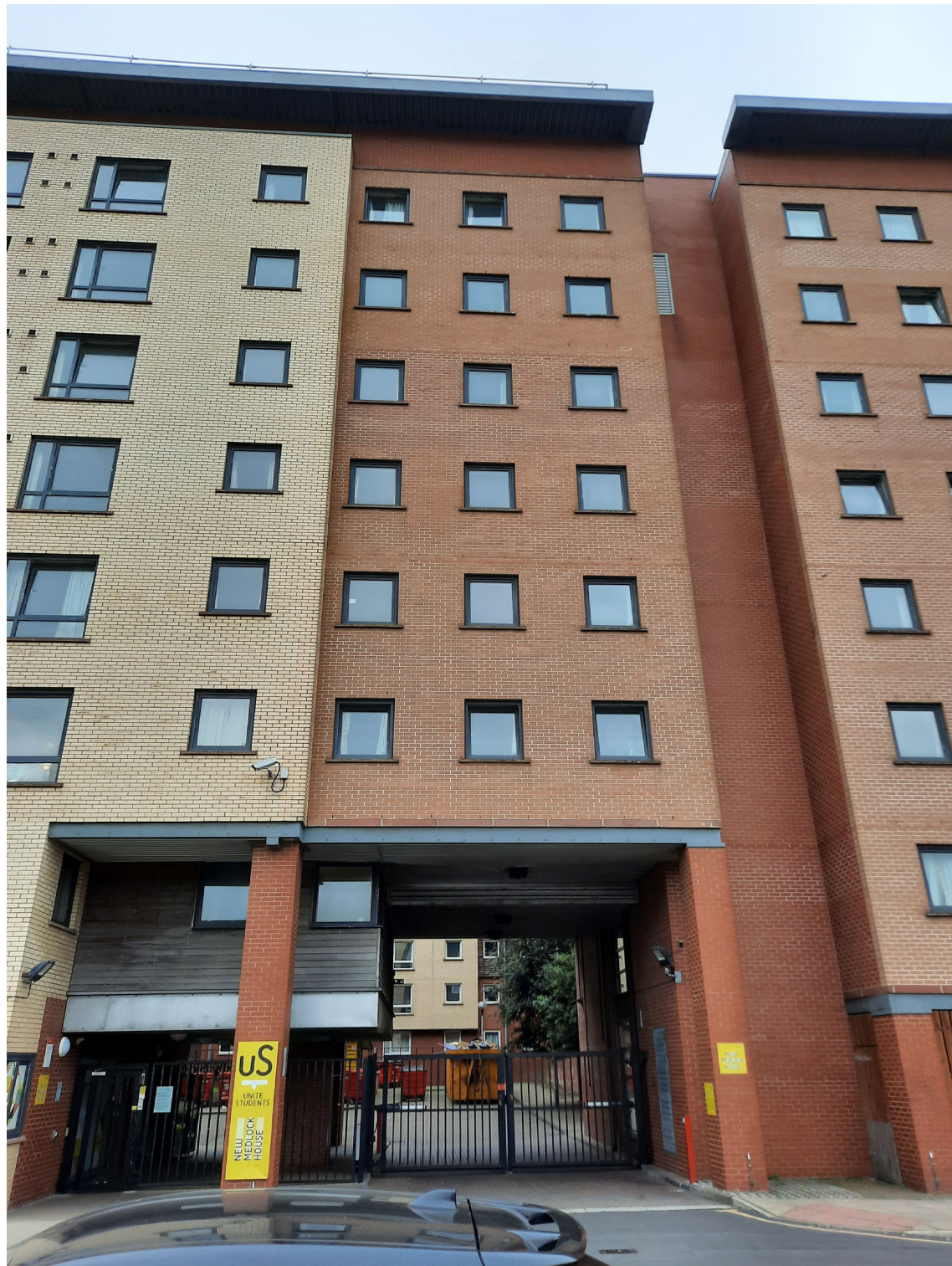
3 Existing North-West (View from Chester Street)
