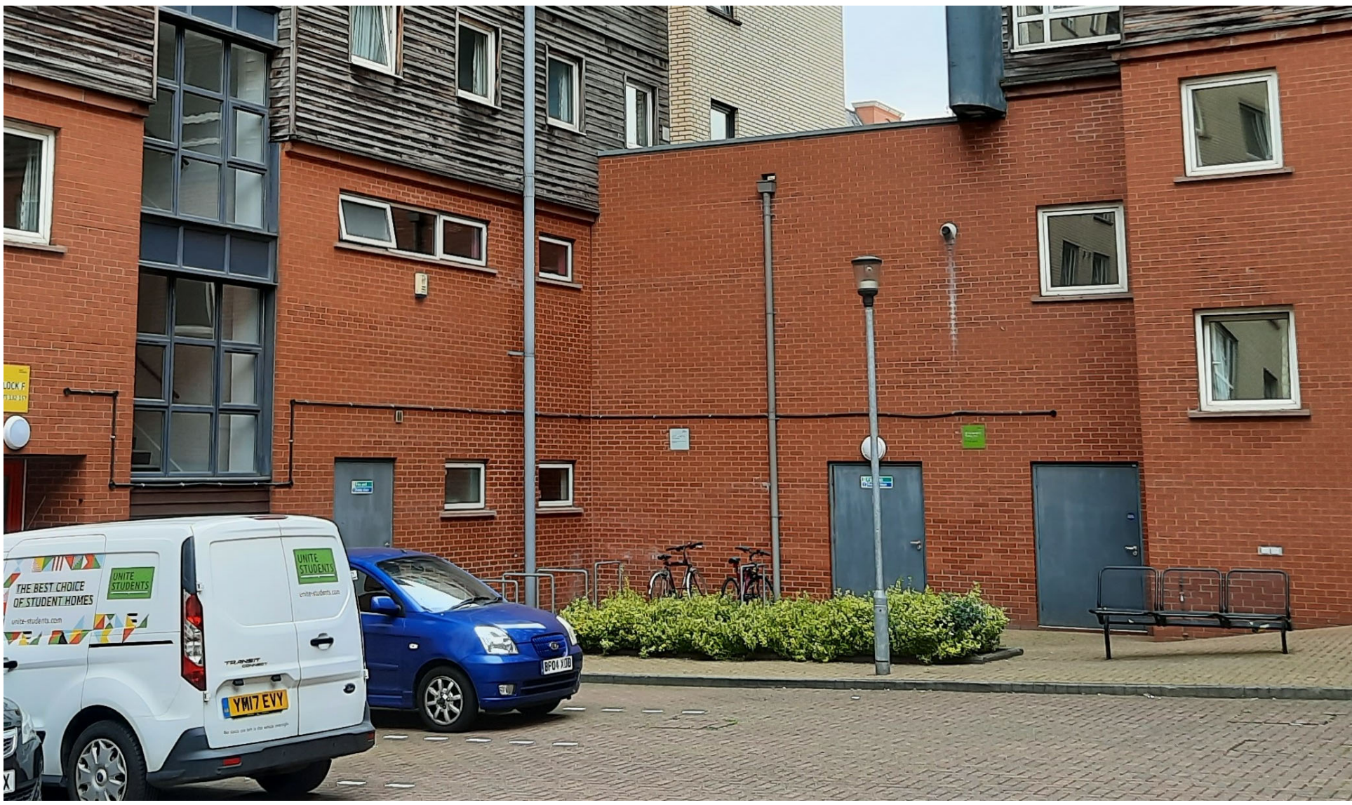
4 Existing North-West & North East (View from Internal Courtyard)
