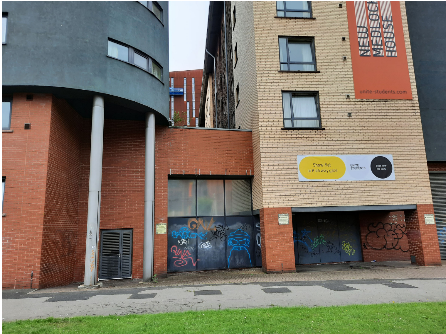
1 Existing North-East (View from Cambridge Street)
