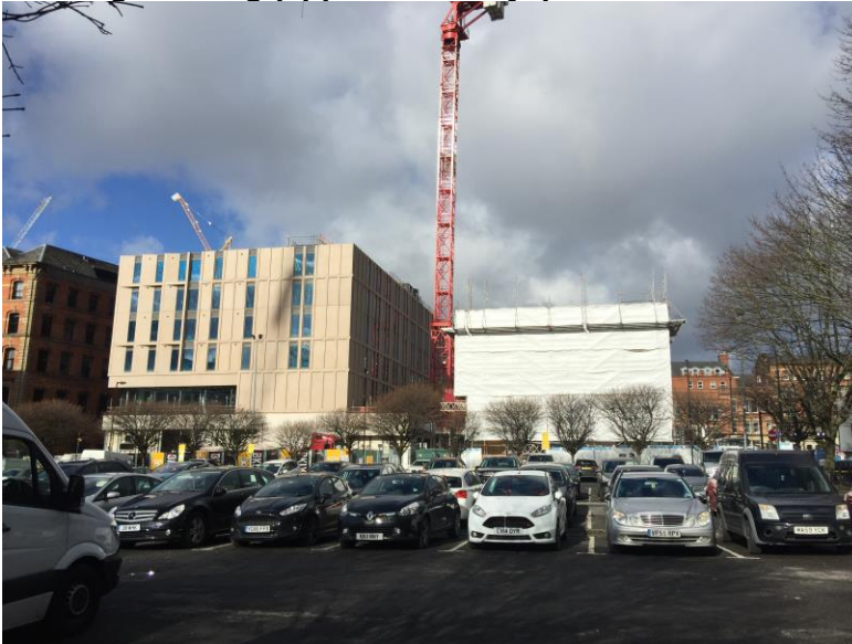
Existing building (approx 5 storeys) March 2019
