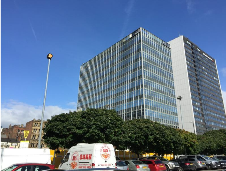
Existing building (12 storeys) October 2017
