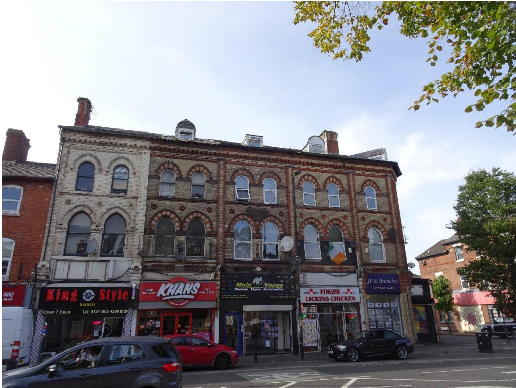
Group of buildings all of the same construction period, although the far left hand building appears that the brickwork has been painted, good quality Tuscan style archways in contrasting brick, indications there have been dormers on all five properties in the past.
