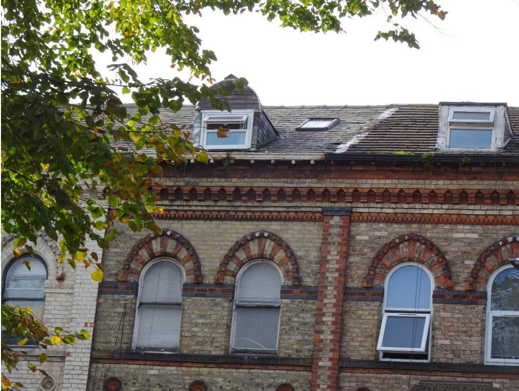
Current dormer detail to property with rooflights to the left and right.
