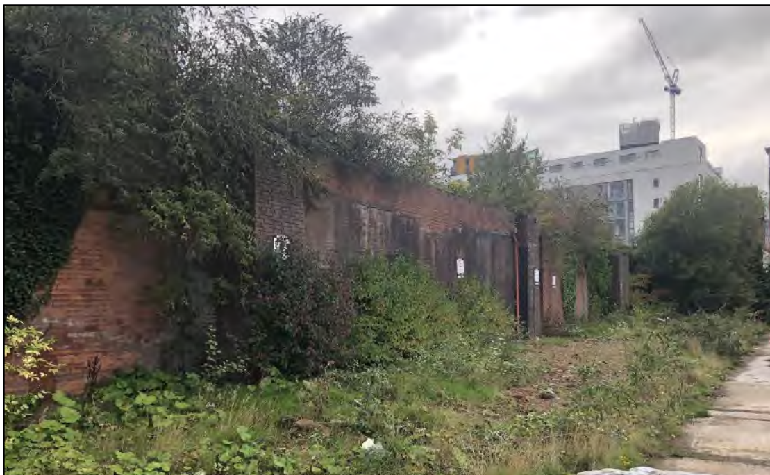
Plate 30: Brick wall along northern boundary of the Site, looking south towards the Site
