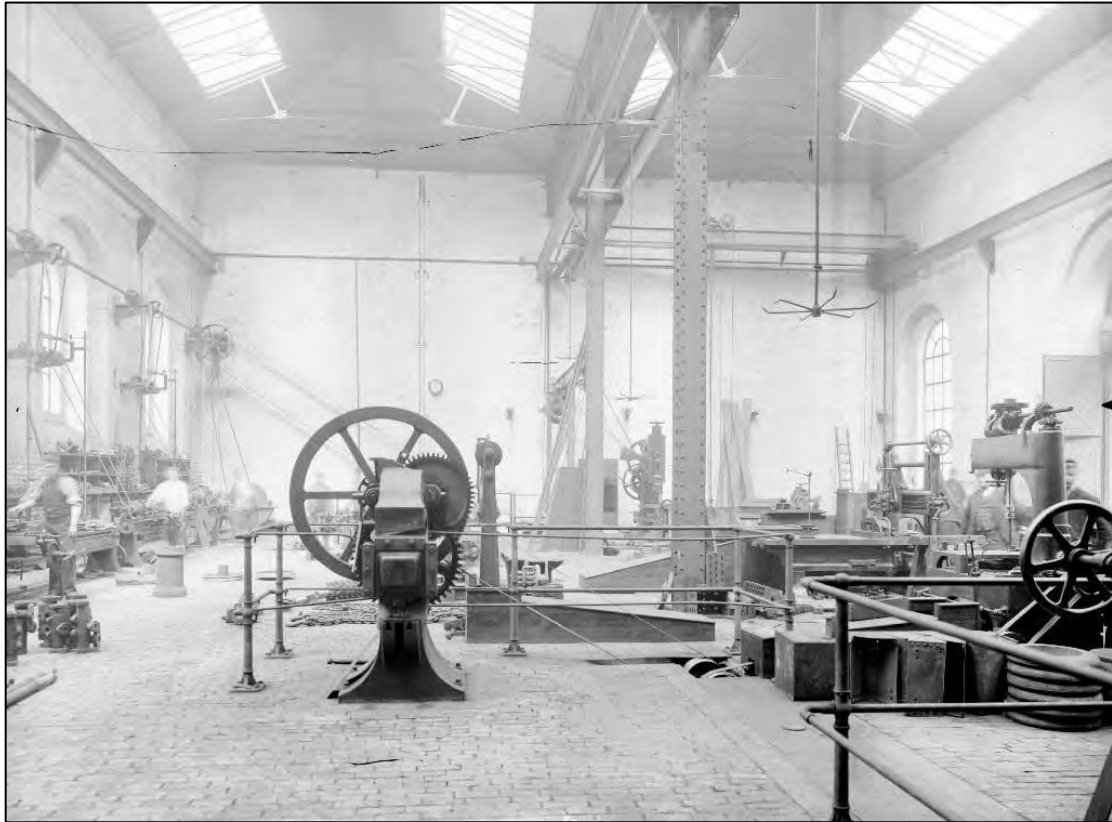
Plate 5: Mechanics shop 1901 Rochdale road gas works
