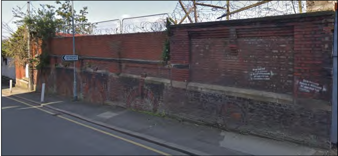
Plate 27: Surviving brick wall in Gould Street, looking east towards the Site
