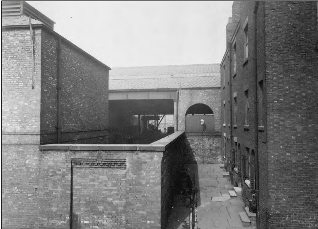
Plate 14: Photograph taken in 1901 showing Gould Street School to the right, the warehouse formerly located within the Site in the background and another building associated with the works to the left
