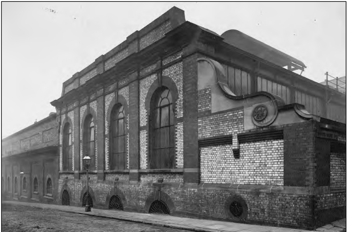
Plate 28: Rochdale Road Gas Works in Gould Street, Manchester 1907
