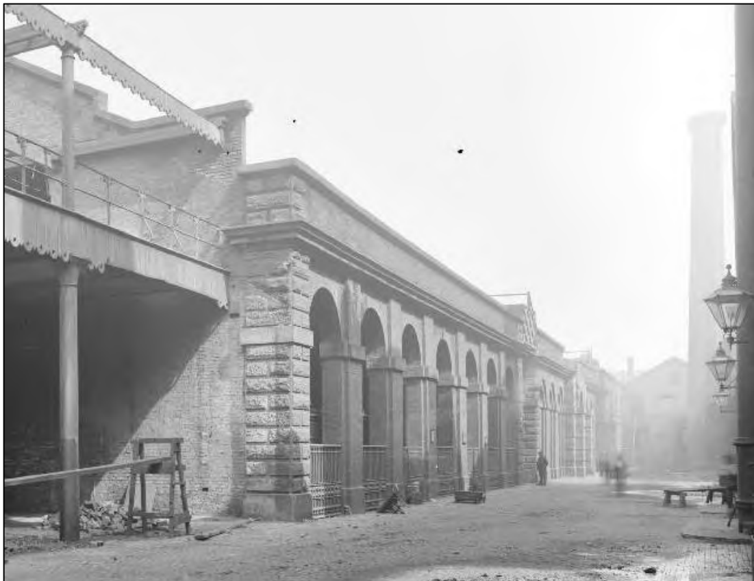
Plate 26: Similar arches within a different part of the gas works shown in photograph dated to 1901
