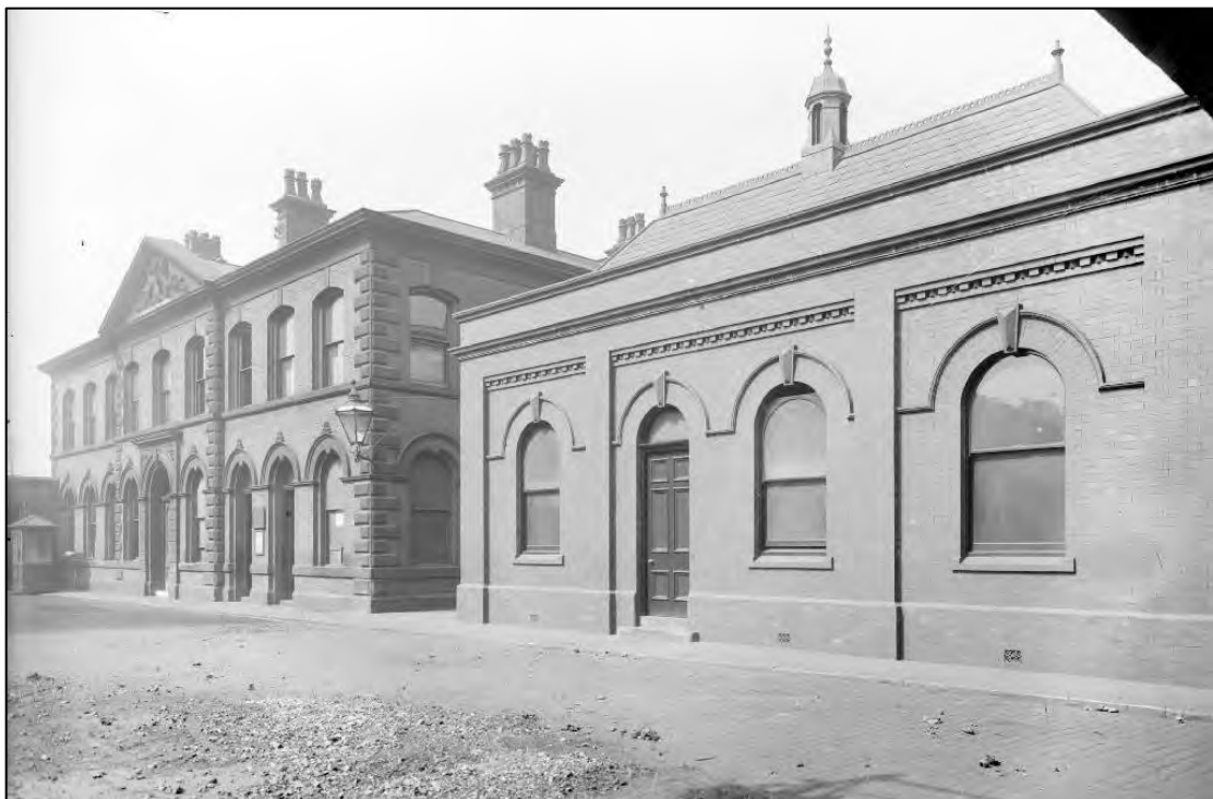
Plate 6: Rochdale Road Gas Works general offices 1901
