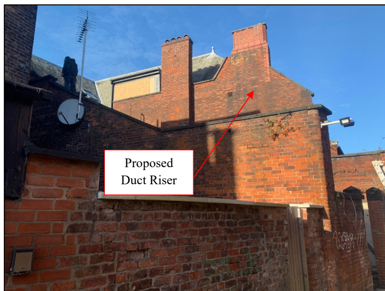
Localised Area to Proposed Mechanical Plant
