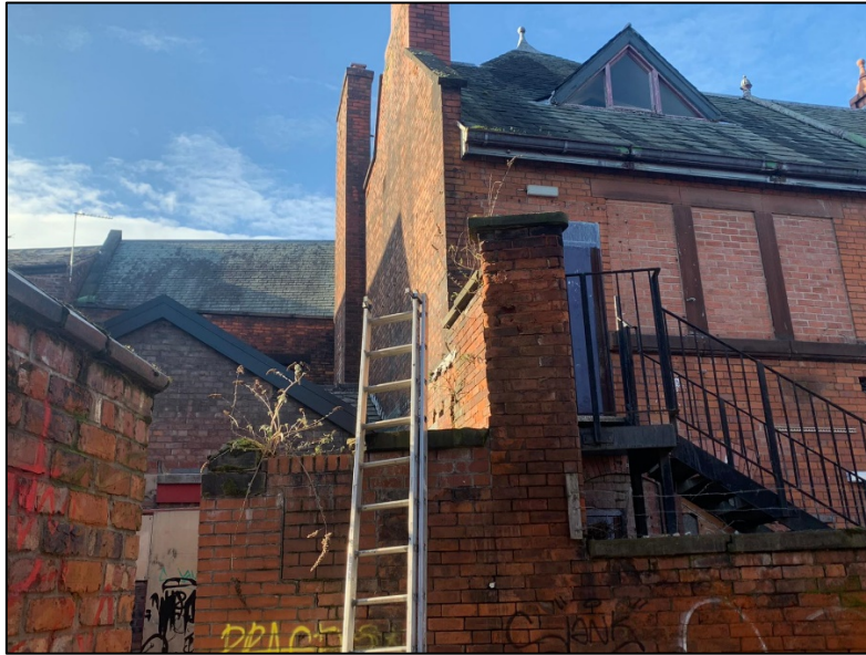
Localised Area to Proposed Mechanical Plant
