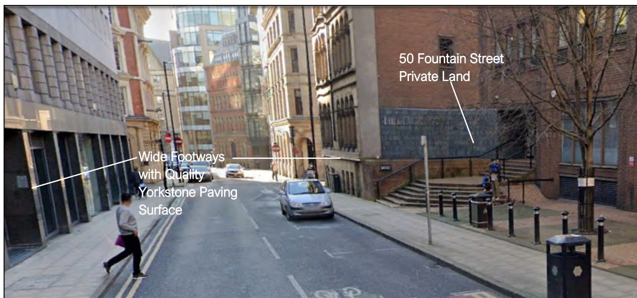
Figure 5.1 Fountain Street Frontage (Looking South) (Google Streetview)
