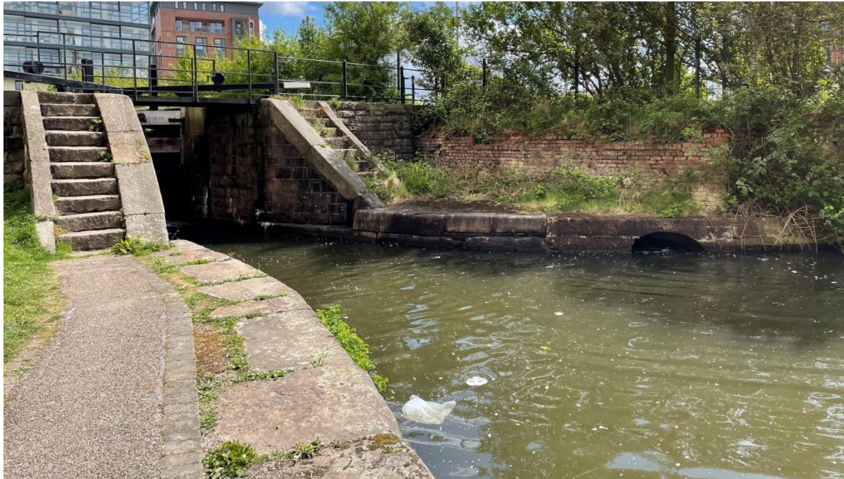
Photograph Five: Lock, retaining walls and paths (looking NE)
