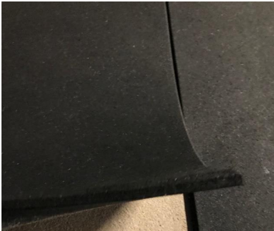
Figure 3 Currently installed rubber gym flooring
