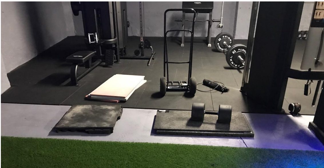
Figure 4 Currently installed rubber gym flooring and other resilient floor types
