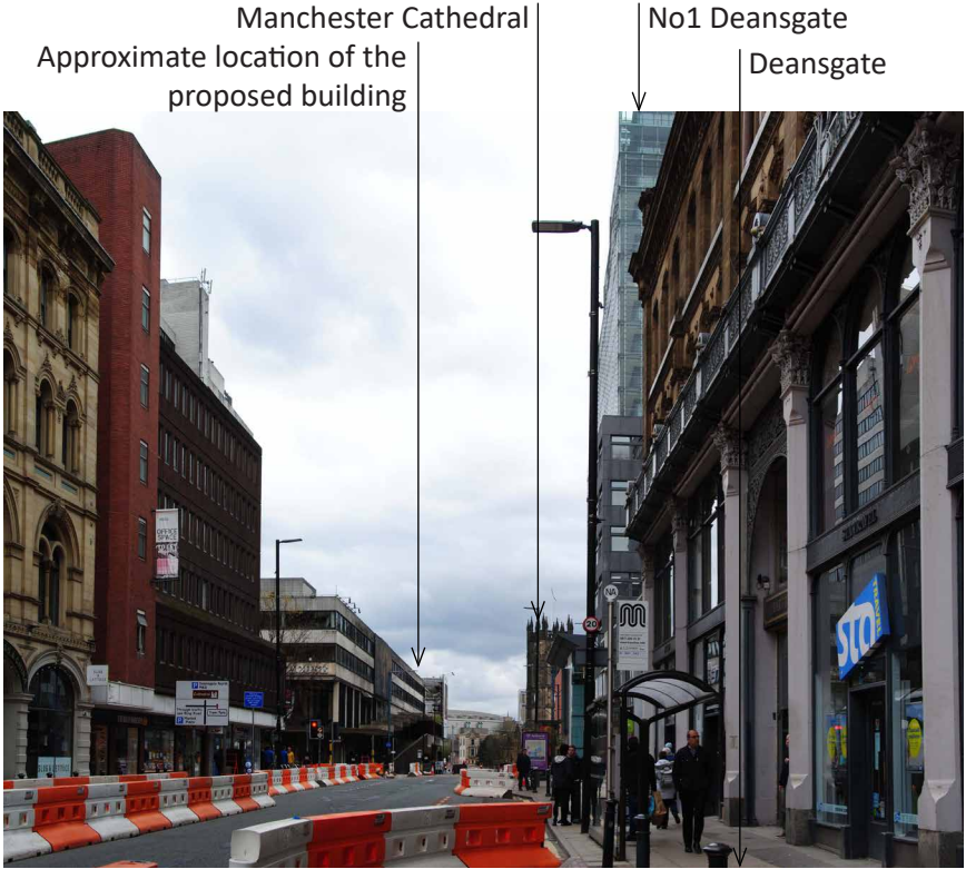
Photograph 6.2 - View from Deansgate, looking north towards the site
