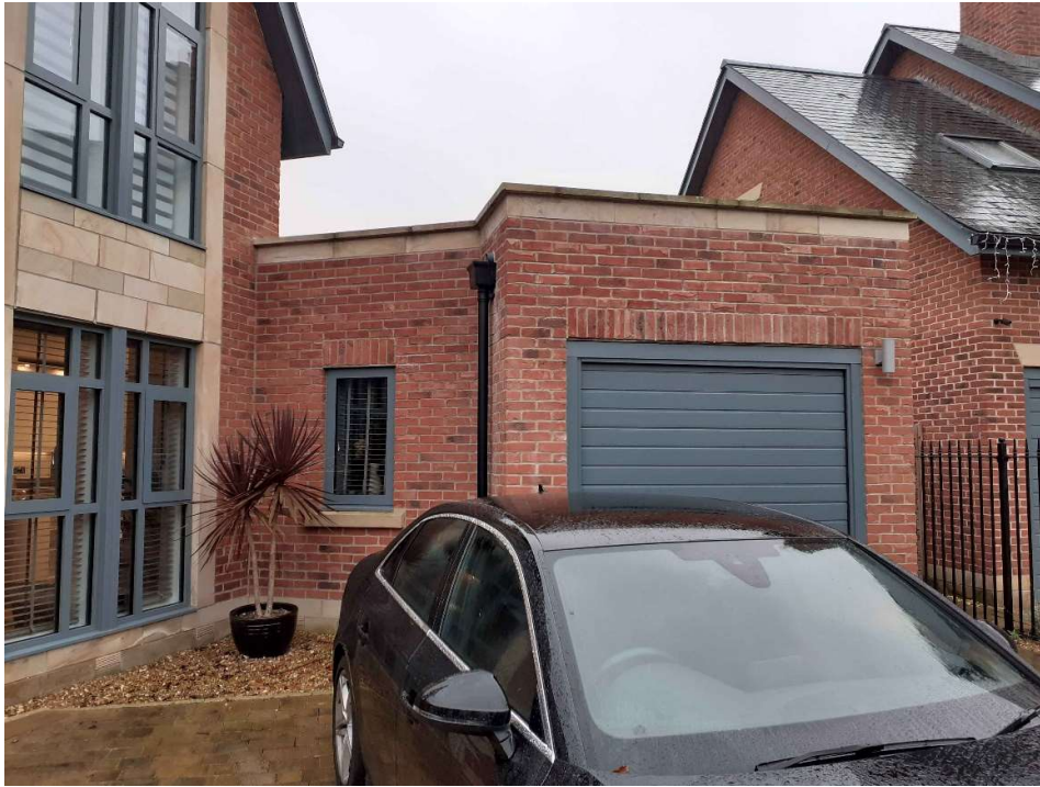
Fig 4. Garage and utility room front façade.
