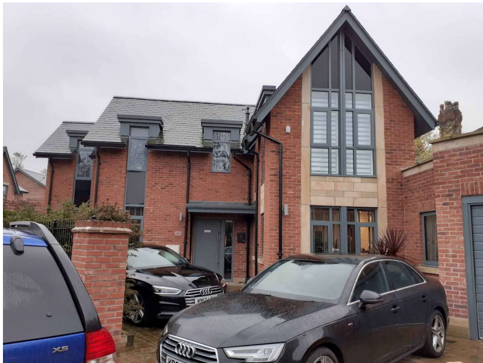
Fig 3. Application Building front façade.
