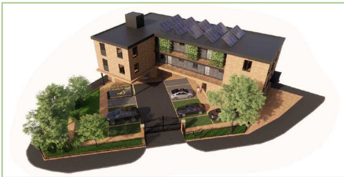
Figure 5.1 – CGI Showing PV Positioning
