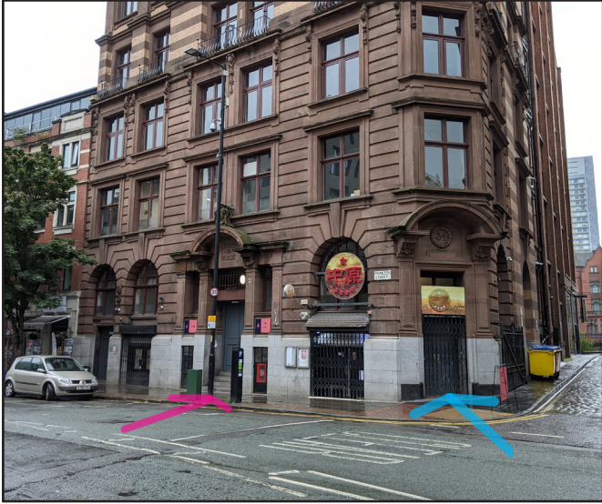
IMAGE 04: View of Manchester House from Princess Street
