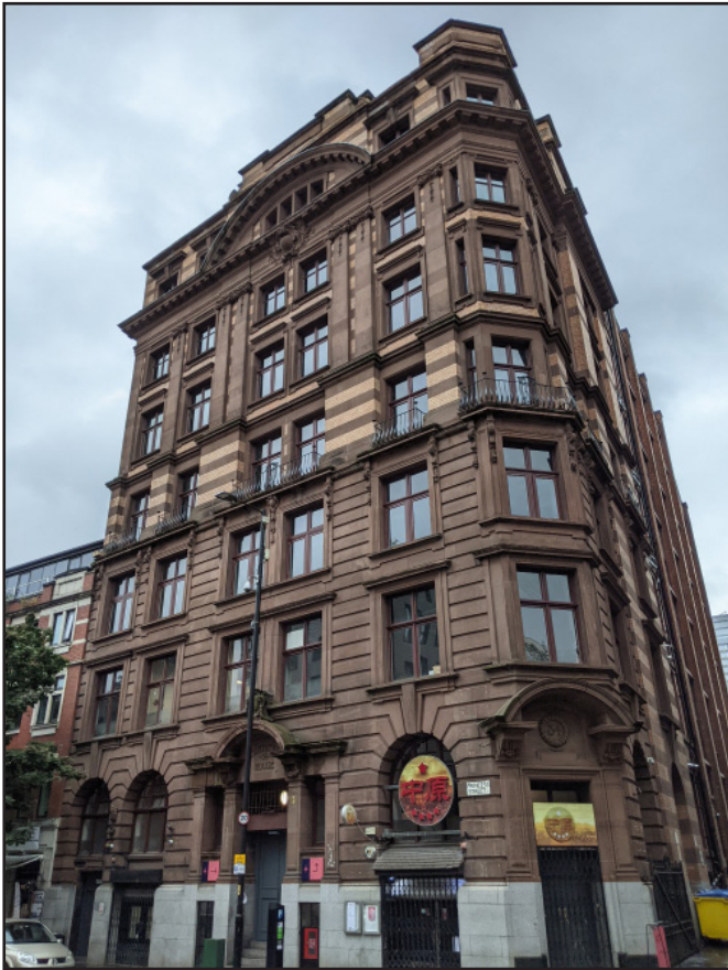
IMAGE 01: View of Manchester House from Princess Street
