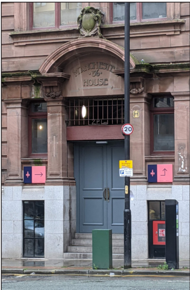
IMAGE 02: Main entrance to Manchester House from Princess Street
