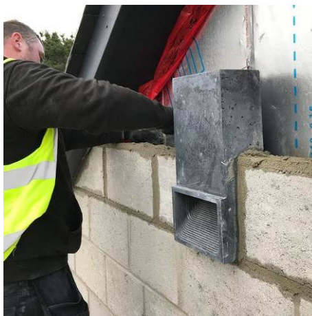
Green and Blue Bat Block/Brick in situ
