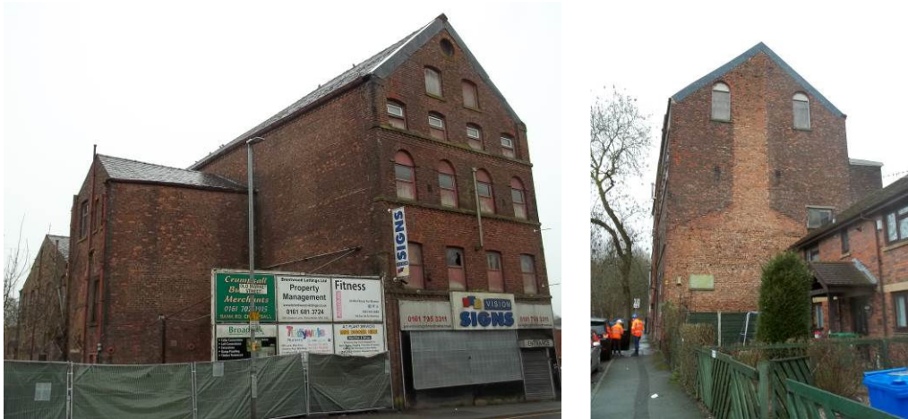
Rear (eastern)/north, and southern elevations
