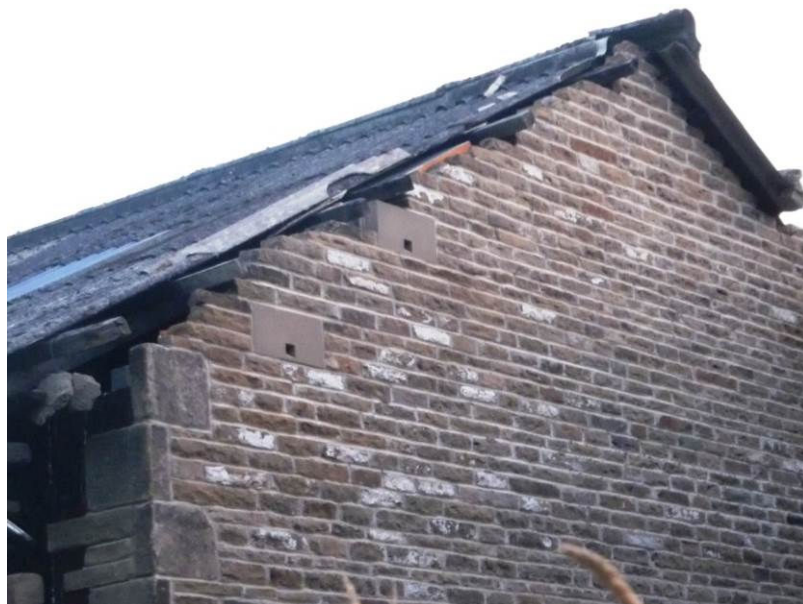
Example of Forticrete boxes in situ
