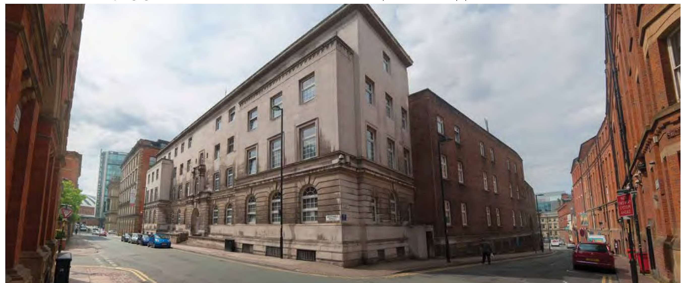
Former Bootle Street Police Station
