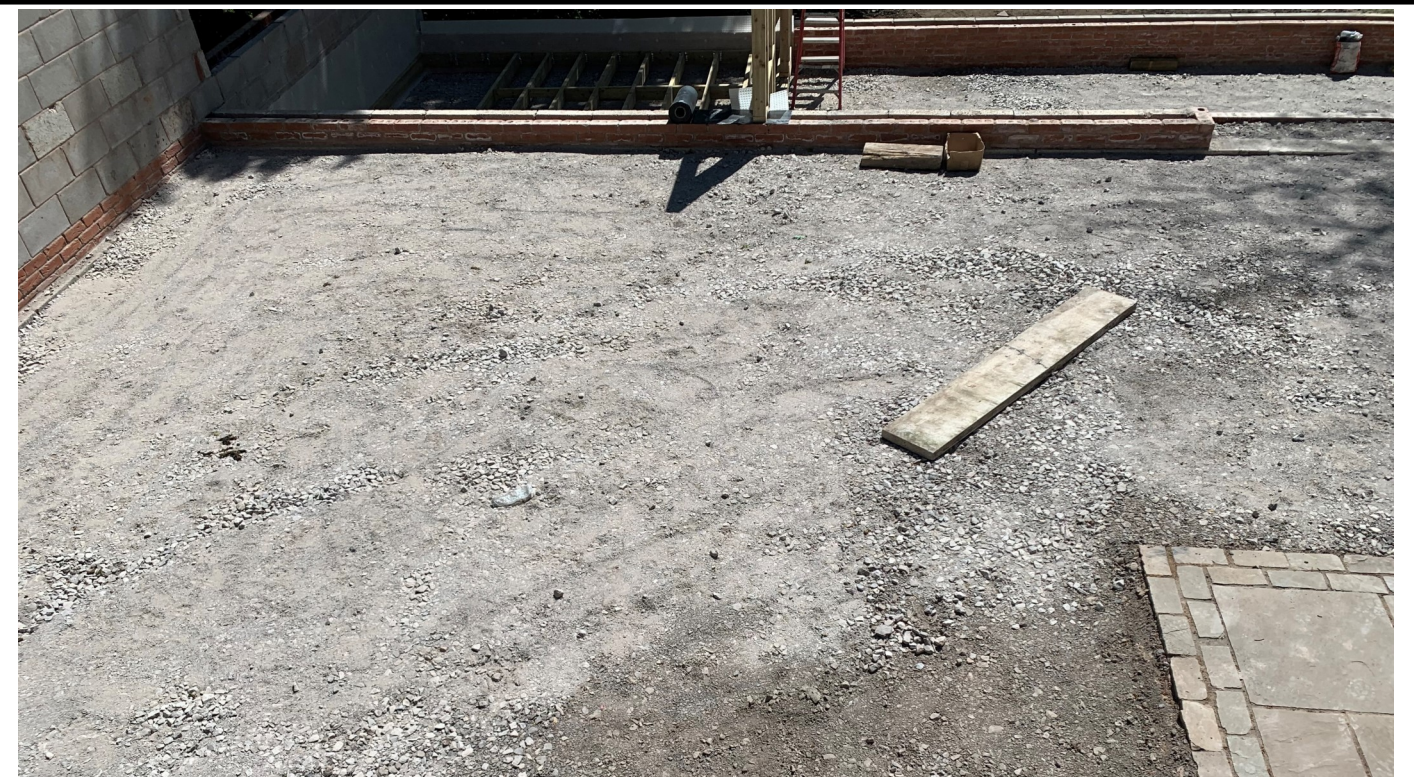
Photo 6: General site photo
