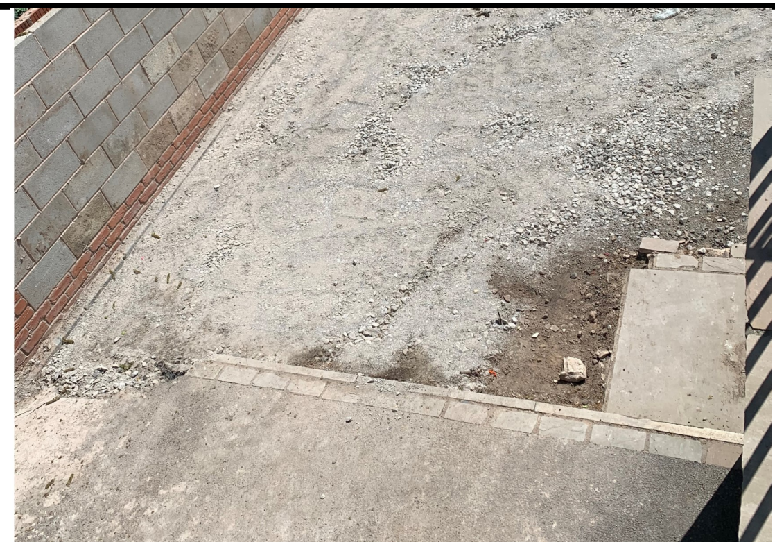
Photo 4: General site photo
