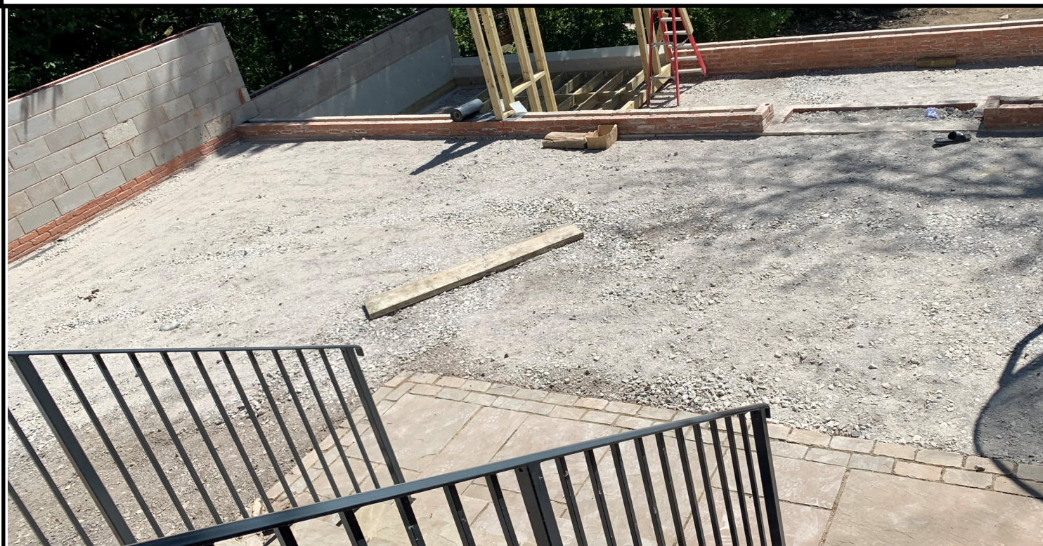
Photo 7: General site photo
