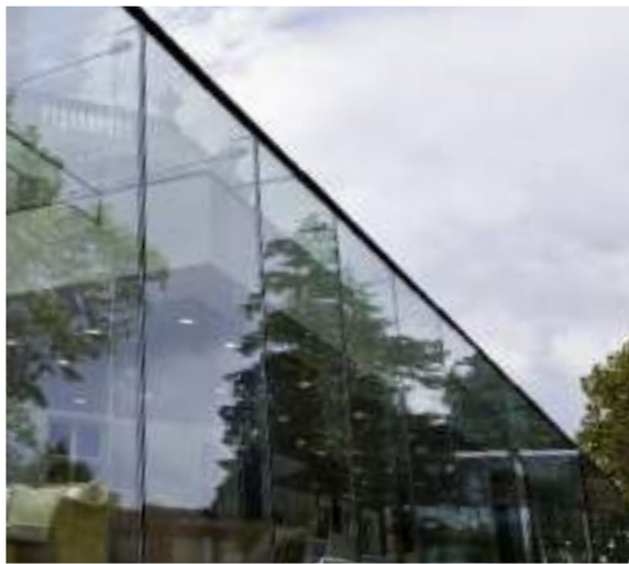
Flameless Glazing, glass to glass corner detail
