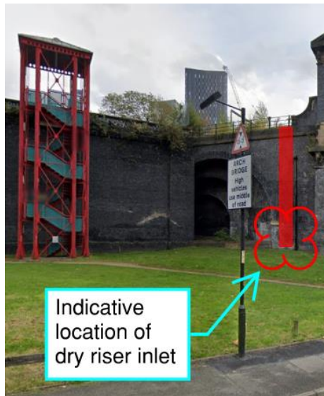
Figure 17: Location of dry riser inlet at street level.
