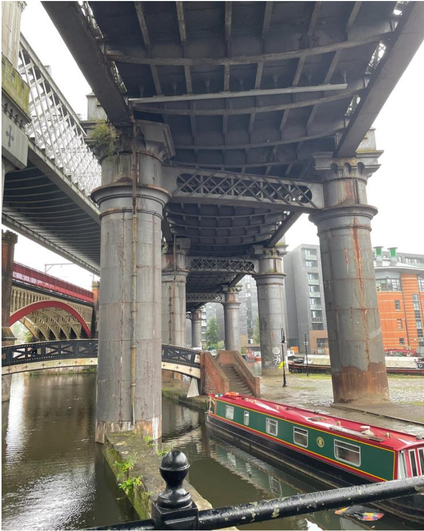
Figure 14: Image showing size of structural columns.
