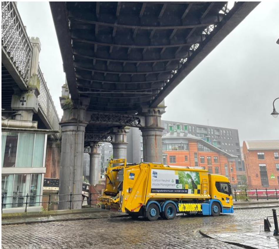
Figure 15: Example of goods vehicle below the viaduct.
