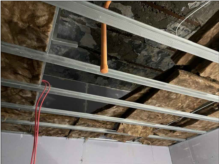
EXISTING BIN STORE CEILING FIFTH FLOOR
