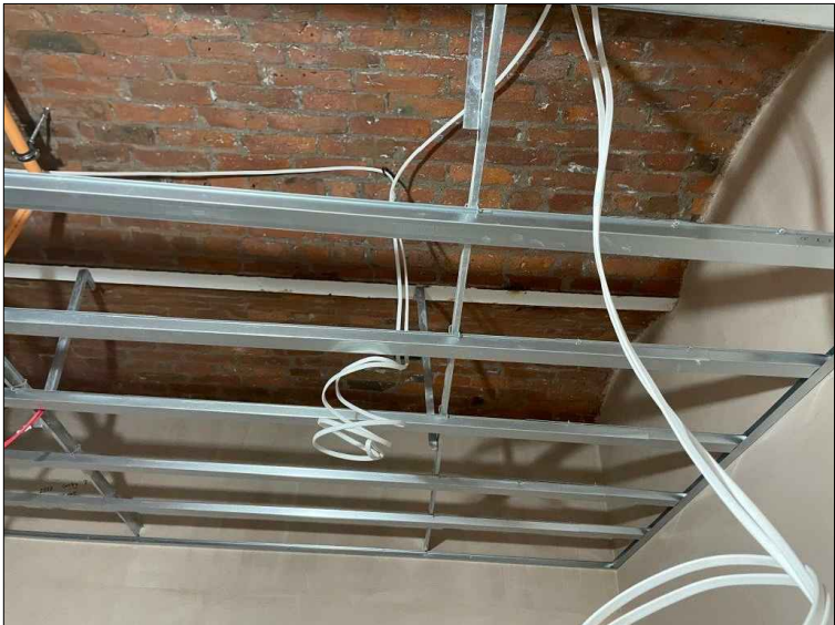
EXISTING BIN STORE CEILING FOURTH FLOOR
