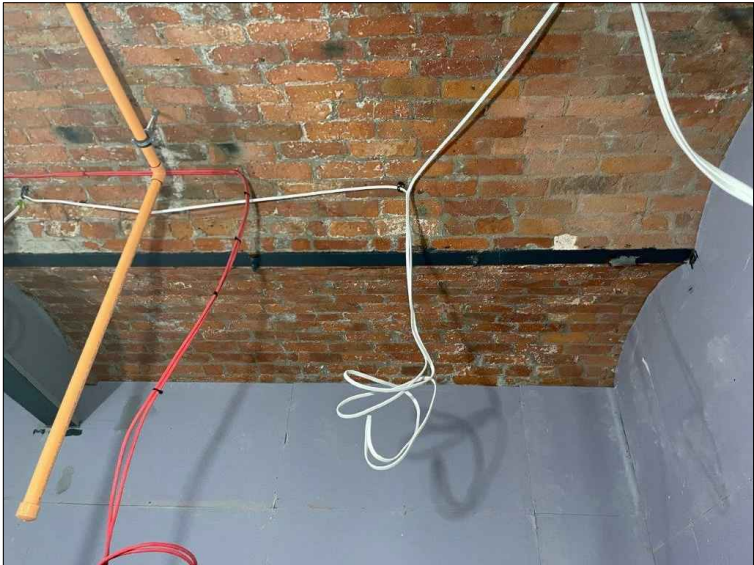
EXISTING BIN STORE CEILING SECOND FLOOR
