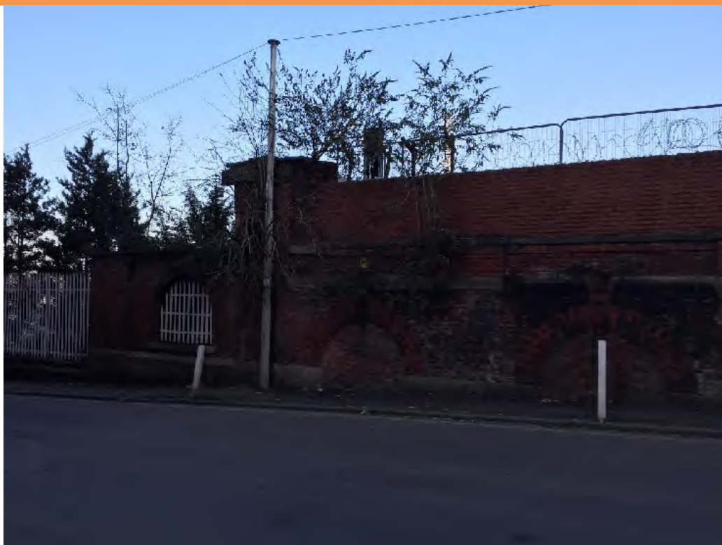
PLATE 4 – VIEW OF SLOPE AND LEVEL CHANGE EXTERNALLY
