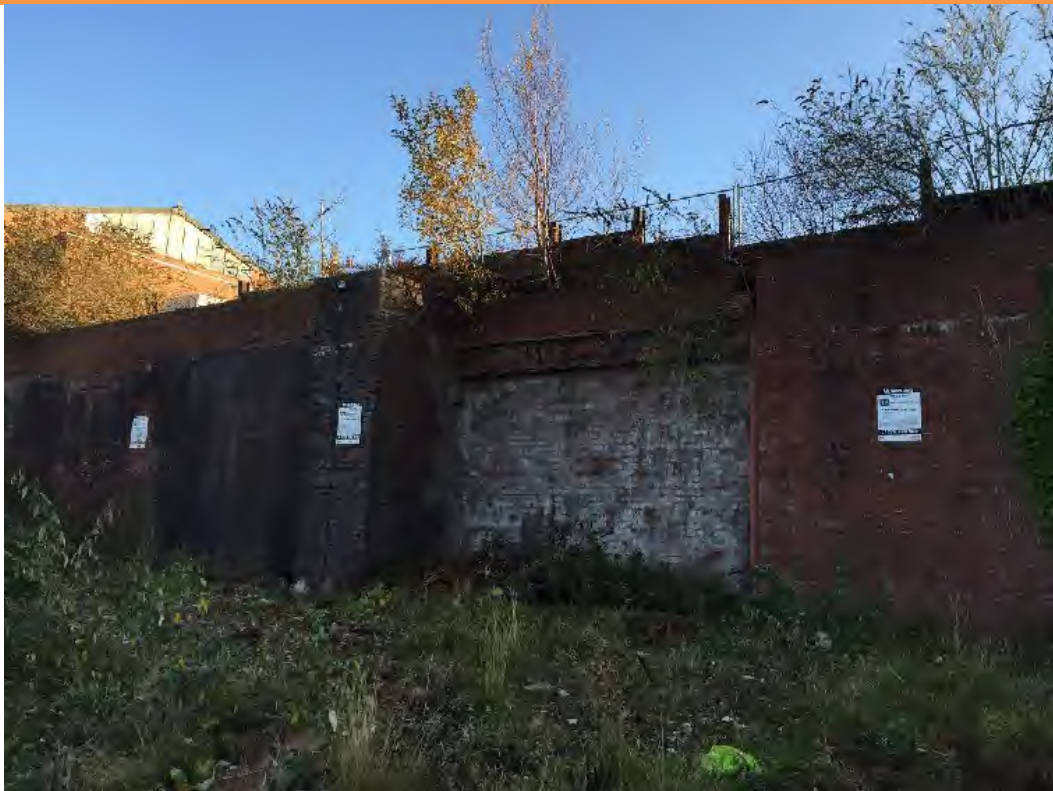
PLATE 3 – VIEW OF RETAINING WALL AT SITE BOUNDARY
