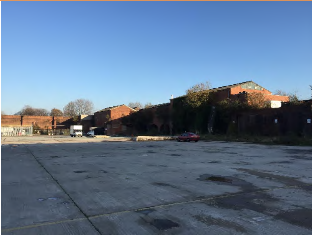
PLATE 1 – VIEW ACROSS SITE
