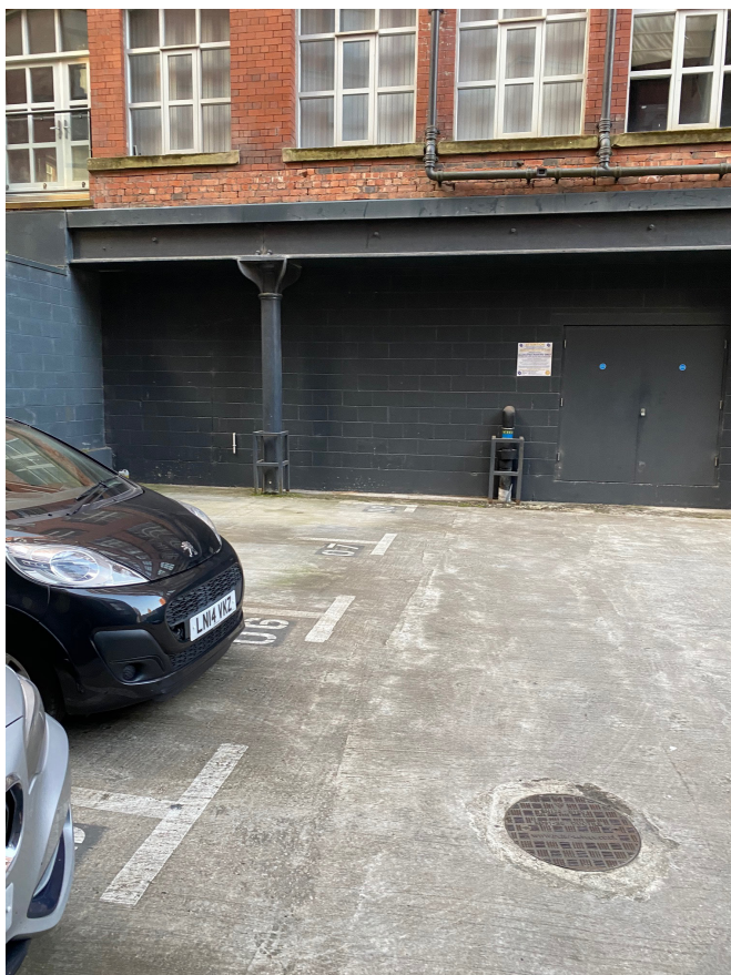
Existing Wall Facing Courtyard
