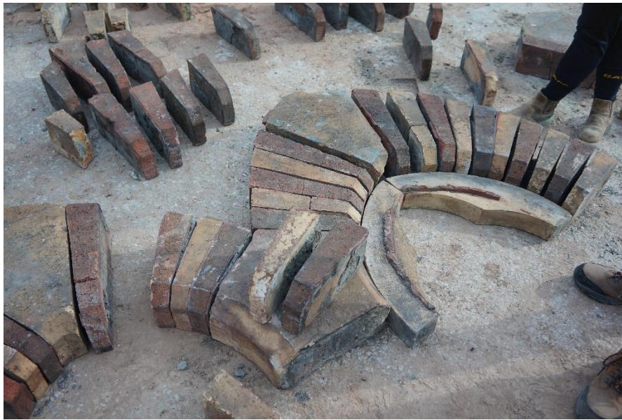
Evidence of abrasive cleaning to polychromatic Voussoirs
