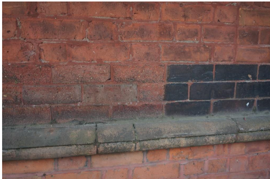
Evidence of previous abrasive cleaning to dark brick banding
