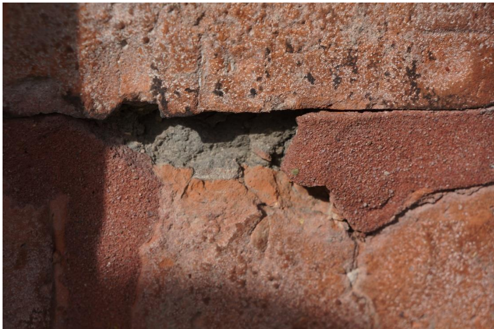
Evidence of original and later mortar samples
