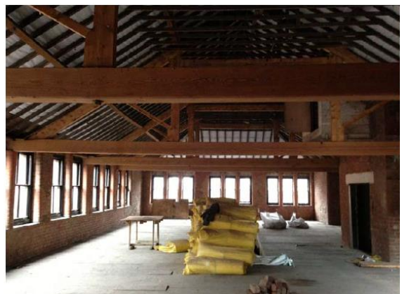
Fig. 10: Interior during conversion works, prior to insertion of internal partitions & mezzanines
