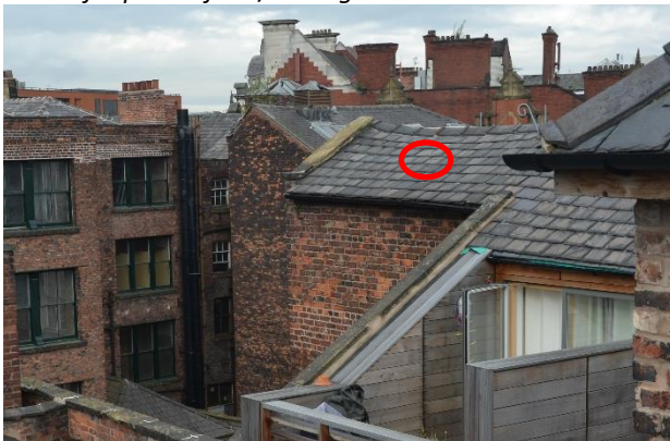
Fig. 11: View towards the rear of apt 3.5, with the location of proposed roof light 1 ringed. (photo taken in 2017)
