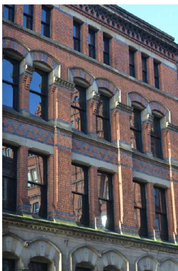
Fig. 6: Architectural detail on the Dale Street elevation
