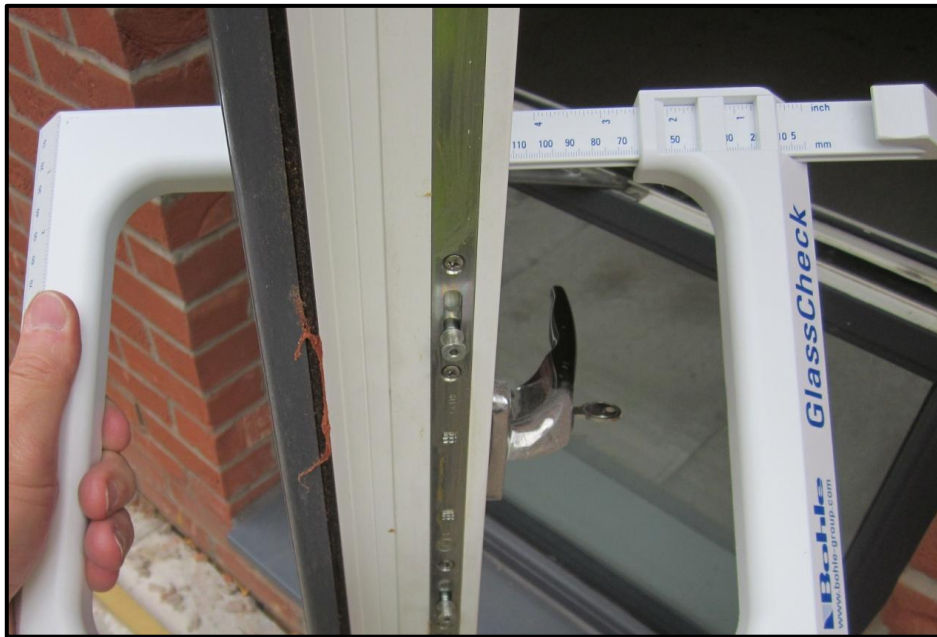
Photograph 3. Measurement of the typical glazing thickness
