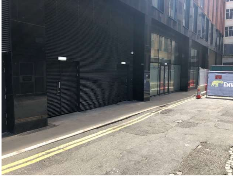
Figure 2: Joiner Street storage access
