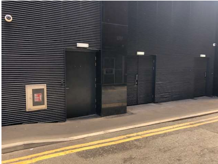
Figure 1: Joiner Street storage access
