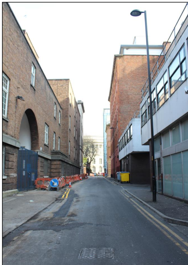
Figure 4 - View along Bootle Street
