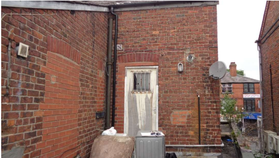
Rear elevation of property (first floor)
