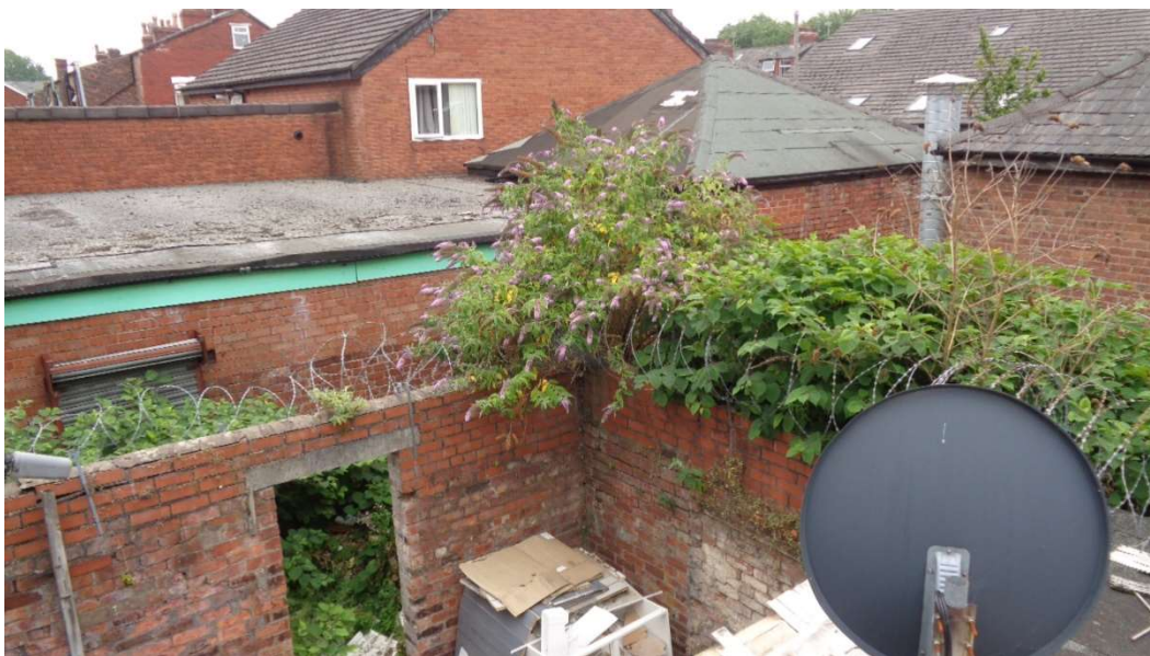
View of rear of property and gated access
