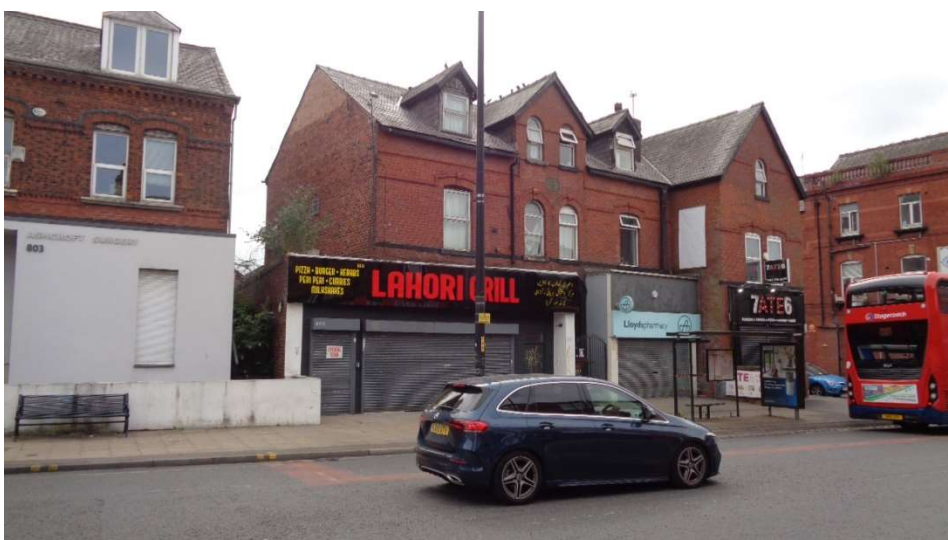
Gable elevation viewed from Stockport Road.
