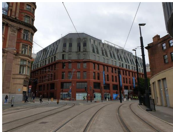
Image 3: View of building from north
