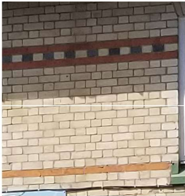
Brickwork to match existing
