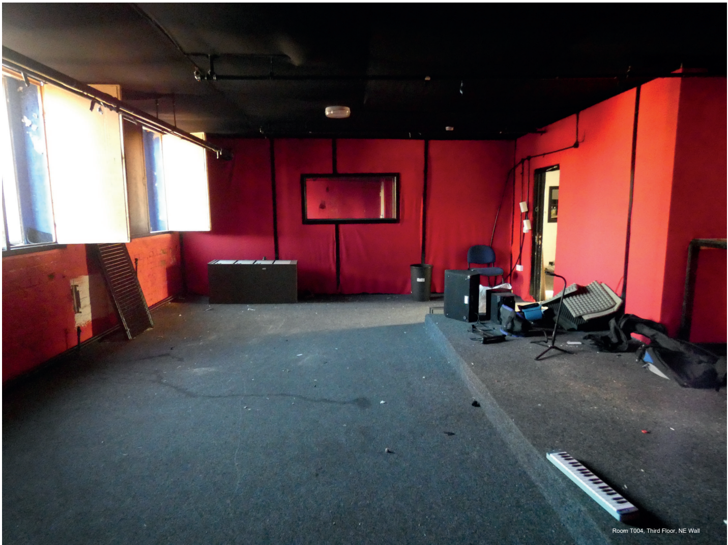
Room T004, Third Floor, NW Wall
