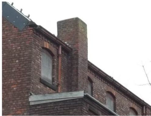
Plate 2. Chimney (eastern elevation) around which bats were seen flying
