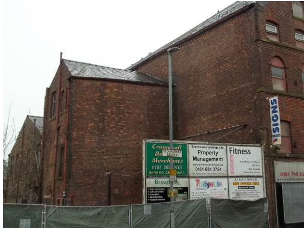
Plate 1. Eastern elevation. Bat seen leaving yard quite close to the building at about mid-height
