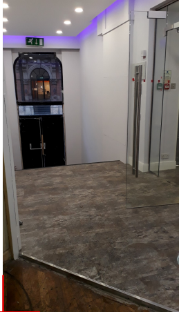
PHOTOGRAPH OF ENTRANCE LOBBY 0/001 SHOWING RETROFIT PLASTERBOARD BULKHEAD CEILINGS WITH INTEGRAL DOWNLIGHTERS
