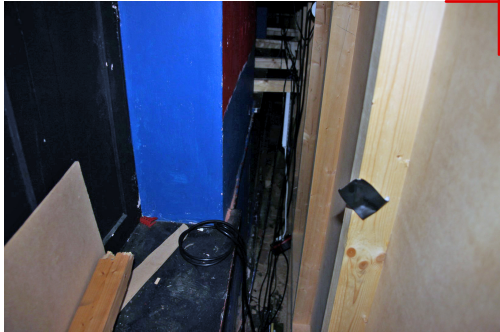
PHOTOGRAPH TAKEN BEHIND THE GENERAL LINING TO GROUND FLOOR NIGHTCLUB WALLS. ALL EXTERNAL WINDOWS ARE BOARDED UP AND INTERNAL WALL FACED LINED WITH OFFSET PLASTERBOARD ON TIMBER STUDWORK.
