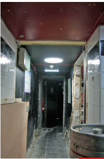
PHOTOGRAPH OF HEAD OF RETROFIT INTERNAL STAIR THAT CONNECTS GROUND AND FIRST FLOOR NIGHTCLUB AREAS. MOST AREAS PLASTERBOARDED AND BOXED IN AND SUBSEQUENTLY PAINTED BLACK FOR NIGHTCLUB USE.
