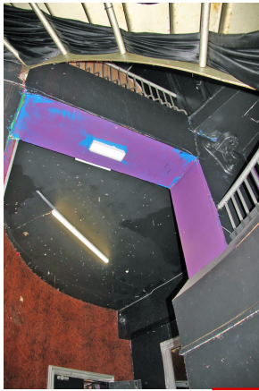
PHOTOGRAPH OF HEAD OF RETROFIT INTERNAL STAIR THAT CONNECTS GROUND AND FIRST FLOOR NIGHTCLUB AREAS. MOST AREAS PLASTERBOARDED AND BOXED IN AND SUBSEQUENTLY PAINTED BLACK FOR NIGHTCLUB USE.
