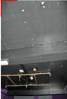
PHOTOGRAPH OF SEATING AREA 0/010 SHOWING RETROFIT PLASTERBOARD CEILING AND BOXING OUT OF TIMBER BEAMS. ALL PAINTED BLACK FOR NIGHTCLUB USE. LIGHTS, ALARMS, INDICATORS AND SPRINKLERS PREDOMINANTLY SURFACE MOUNTED.
