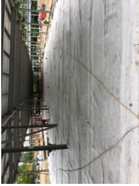
Vent mat connected to perimeter T piece
