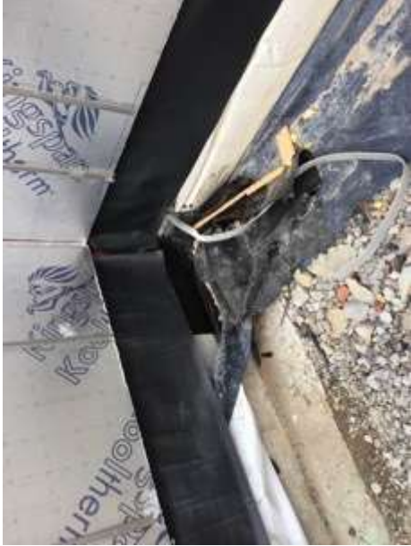
Stanchion seal using SAGM
