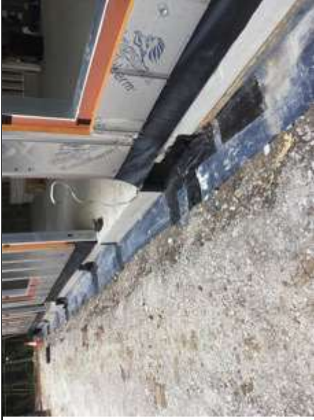
Perimeter edge and stanchions sealed
