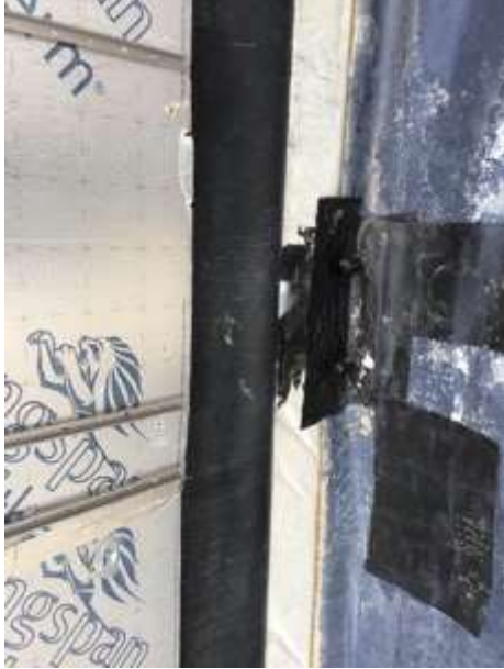
Stanchion seal using SAGM
