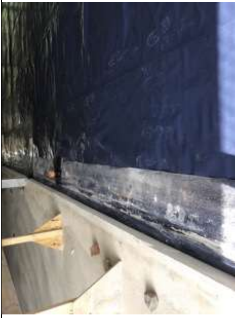
Joint to previously installed membrane
