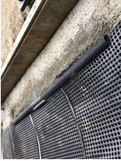
Vent mat joining to perimeter T piece
