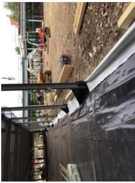
SAGM being pick tested around a stanchion
