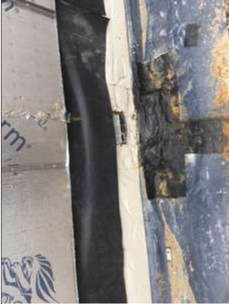
Stanchion seal using SAGM
