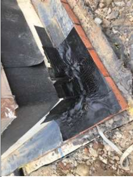
Perimeter corner repair
