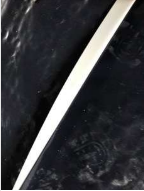
Sealed double sided butyl tape membrane joint
