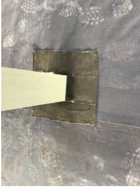
Pipe seal using SAGM
