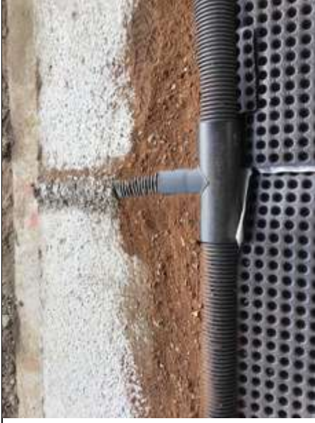
"T" piece with slotted pipe
