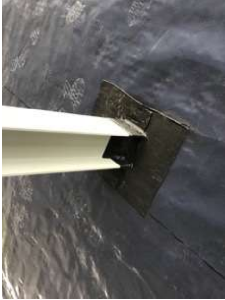
Sealed stanchion detail
