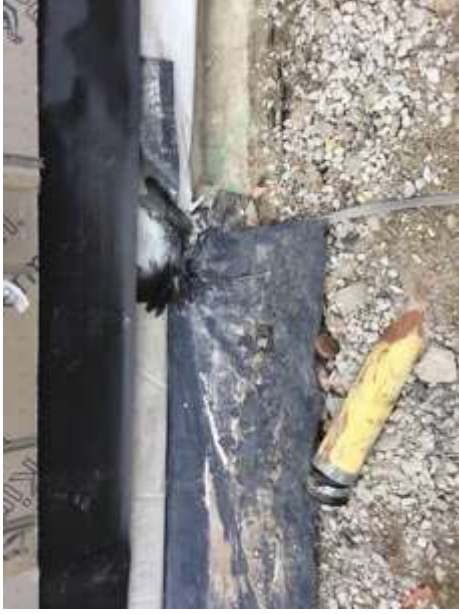
Perimeter edge and stanchions sealed
