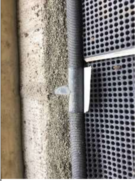
Vent mat joining to perimeter T piece
