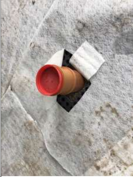
Venting cut around pipe penetration
