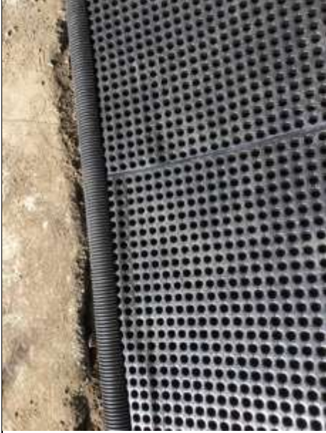
Vent mat inserted into slotted collection pipe
