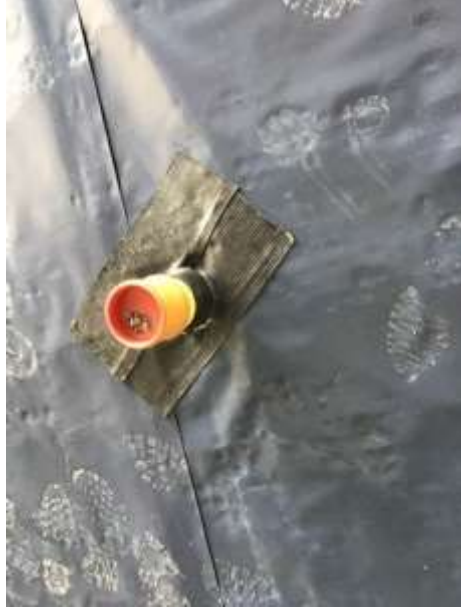
Stanchion seal using SAGM
