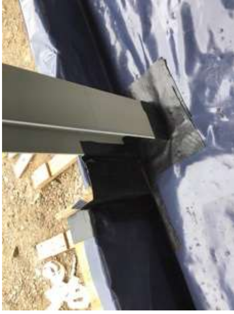
Sealed pipe penetration
