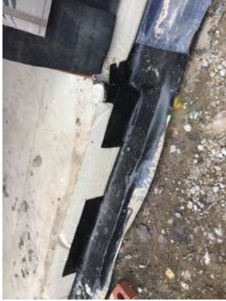
Perimeter corner repair
