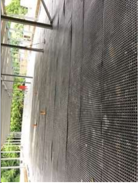
Full venting installation
