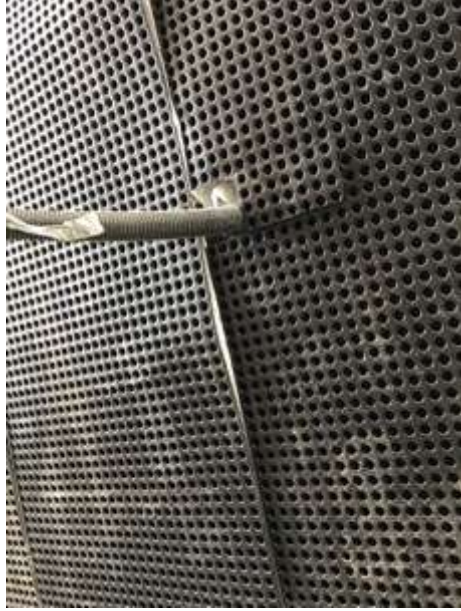
Vent mat inserted into slotted collection pipe
