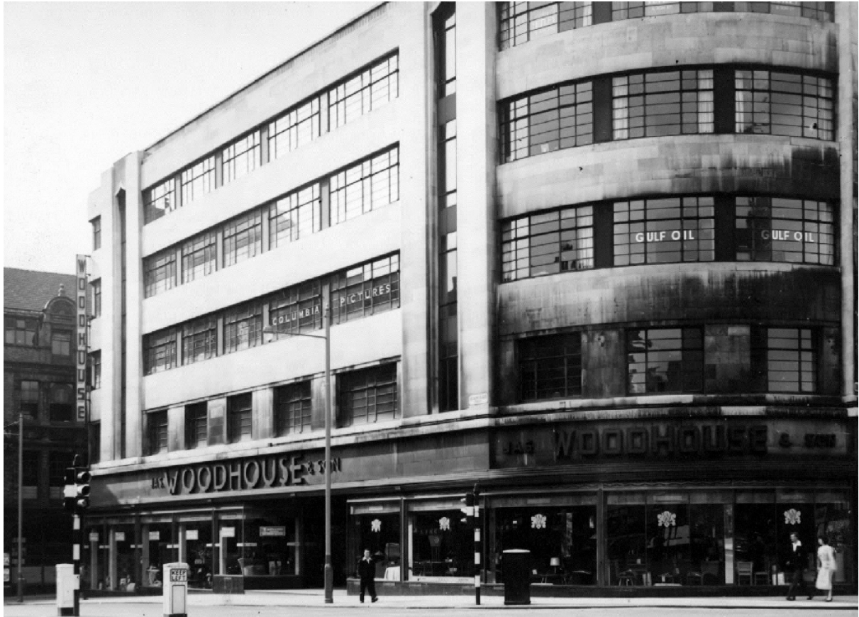
Figure 10: 1956 Blackfriars corner of Deansgate – Woodhouse and Sons Building
