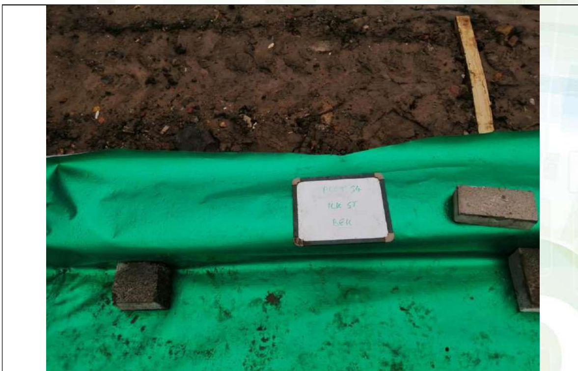
Photograph 8: Validation of Gas Membrane Installation
