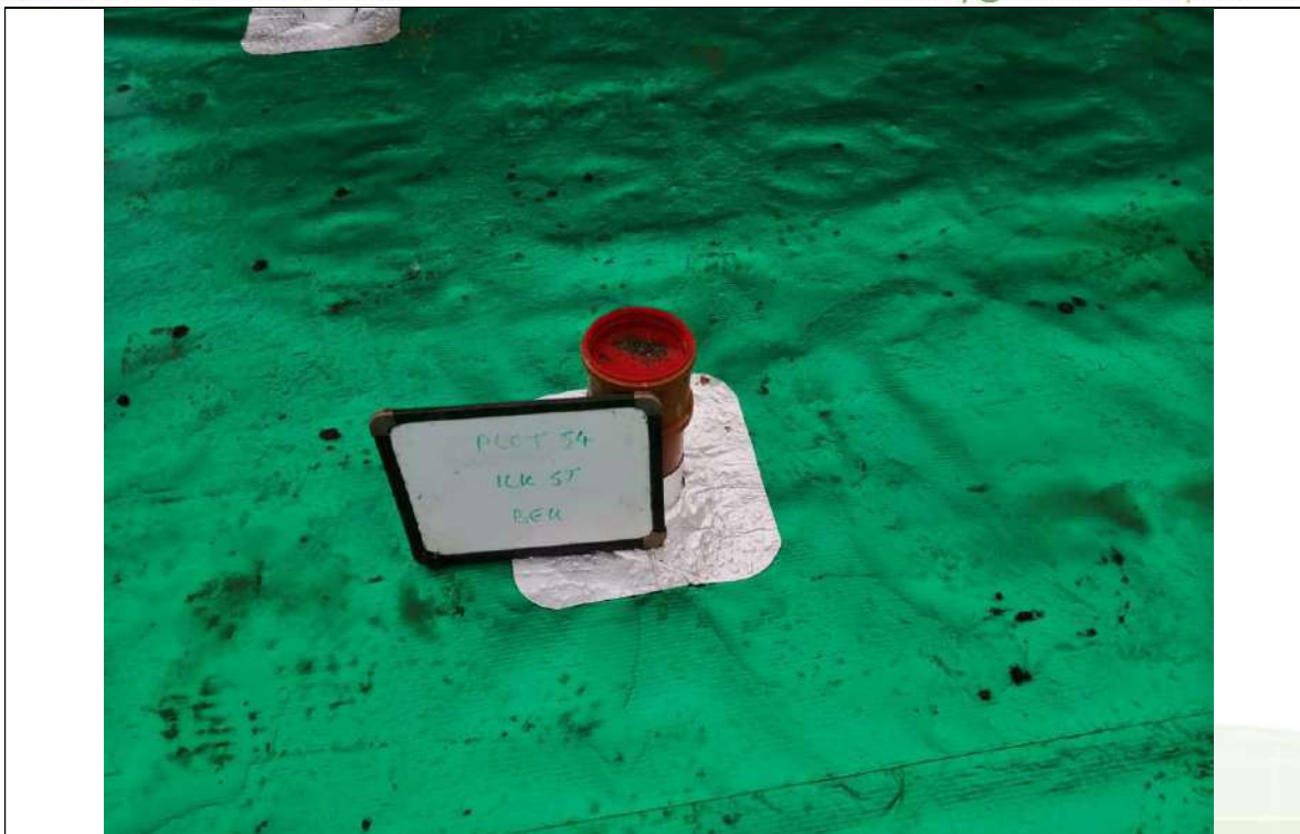
Photograph 7: Validation of Gas Membrane Installation
