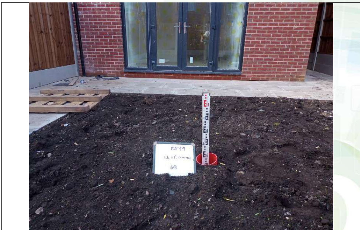
Photograph 2: Validation of Garden Capping Thickness
