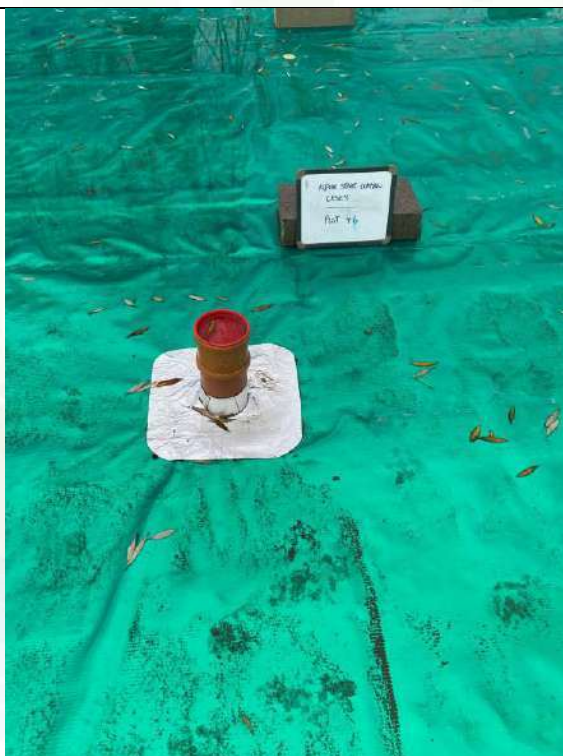
Photograph 6: Validation of Gas Membrane Installation
