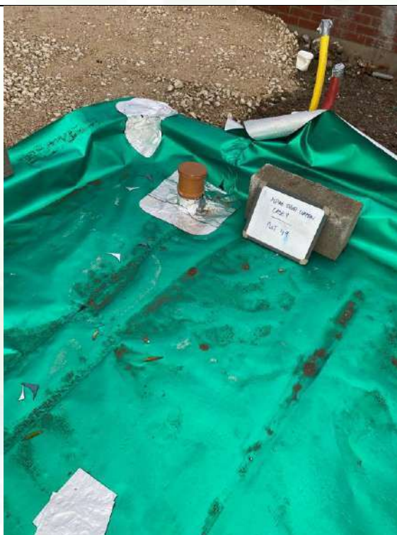
Photograph 6: Validation of Gas Membrane Installation
