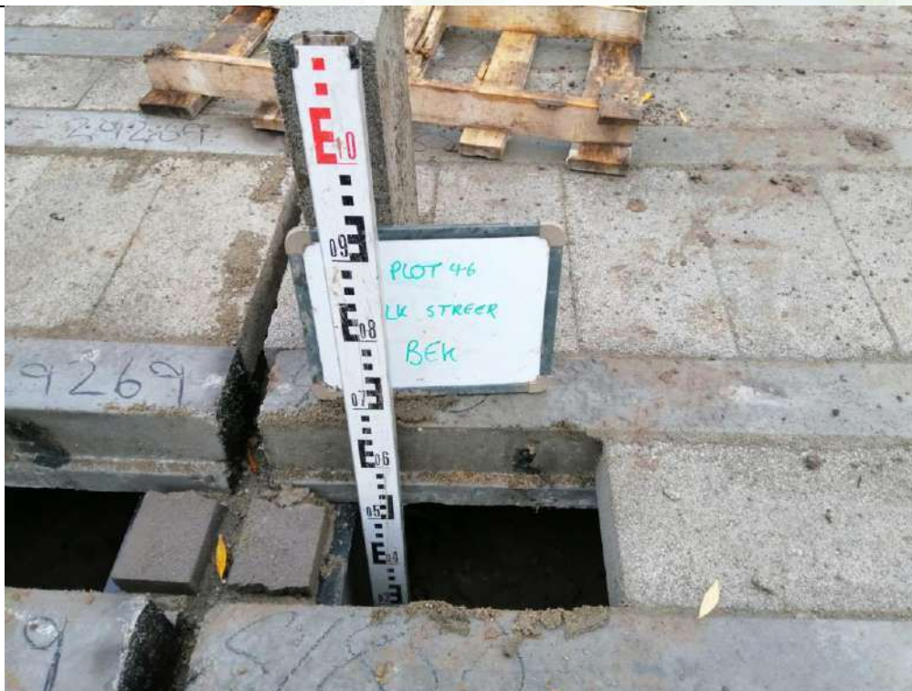
Photograph 4: Validation of Sub-Floor Void Space (min 150 mm)
