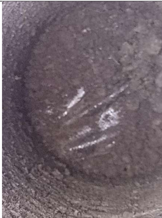
Photograph 3: Validation of Geotextile Membrane
