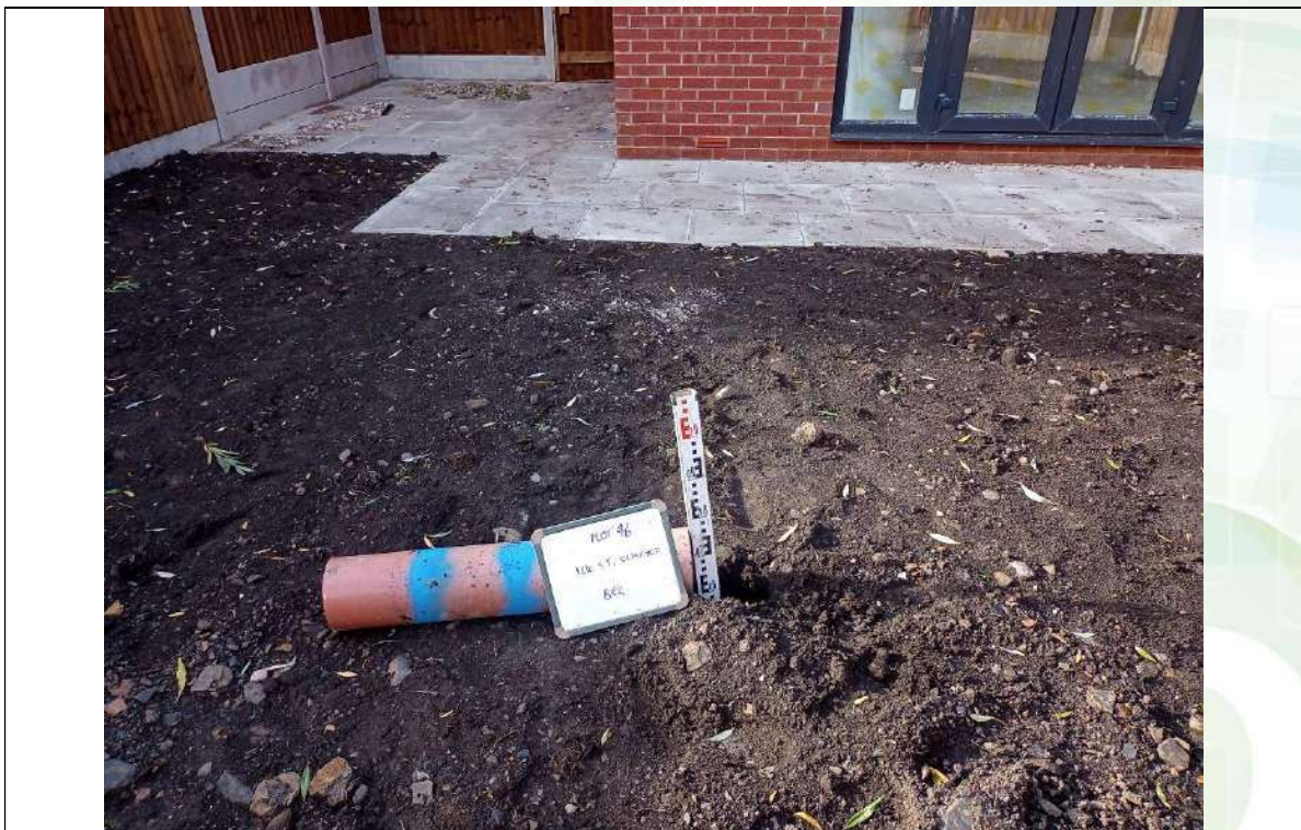
Photograph 2: Validation of Garden Capping Thickness
