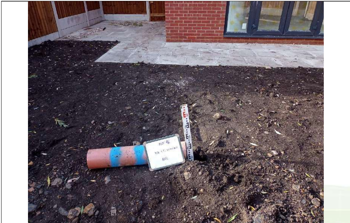
Photograph 1: Validation of Garden Capping Thickness
