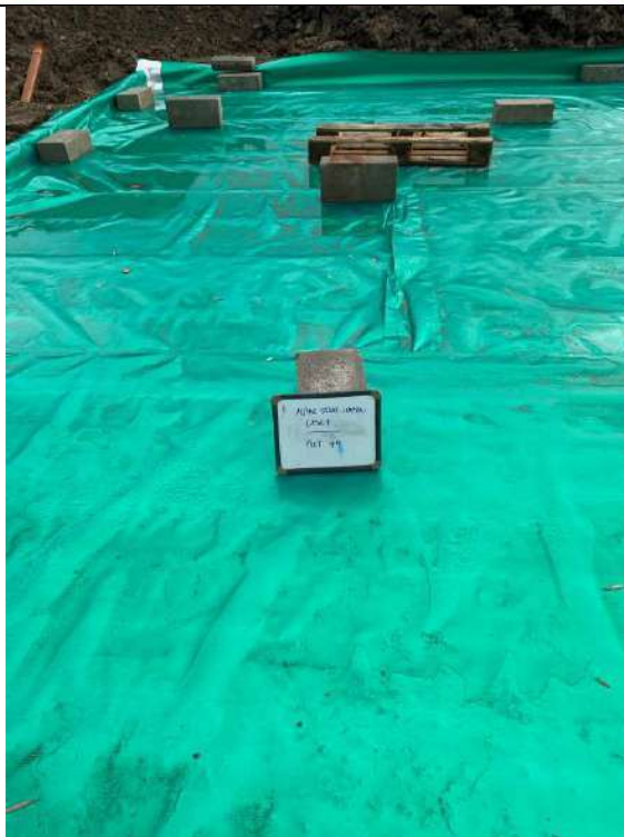
Photograph 5: Validation of Gas Membrane Installation
