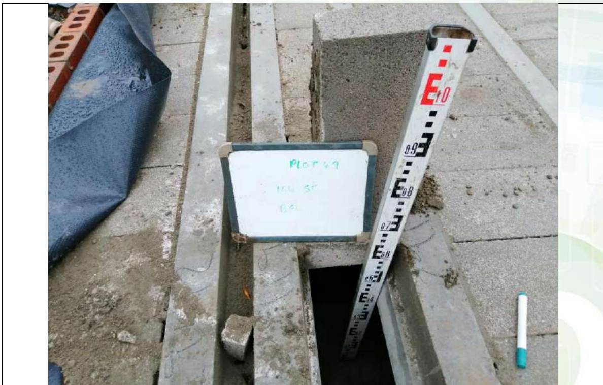
Photograph 4: Validation of Sub-Floor Void Space (min 150 mm)
