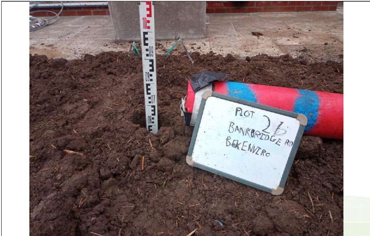
Photograph 1: Validation of Garden Capping Thickness
