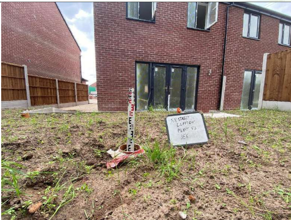
Photograph 2: Validation of Garden Capping Thickness (Plot 54, not 53)
