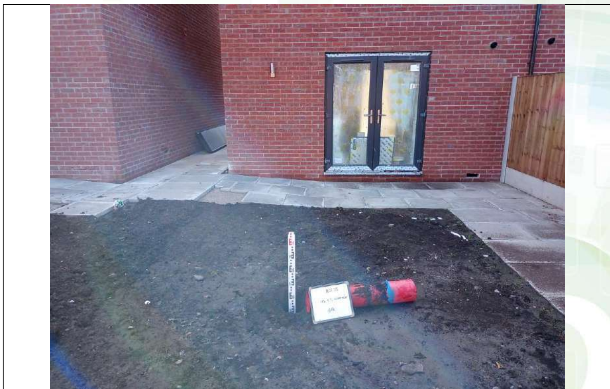
Photograph 2: Validation of Garden Capping Thickness
