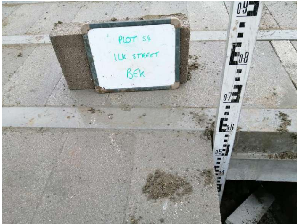
Photograph 3: Validation of Sub-Floor Void Space (min 150 mm)
