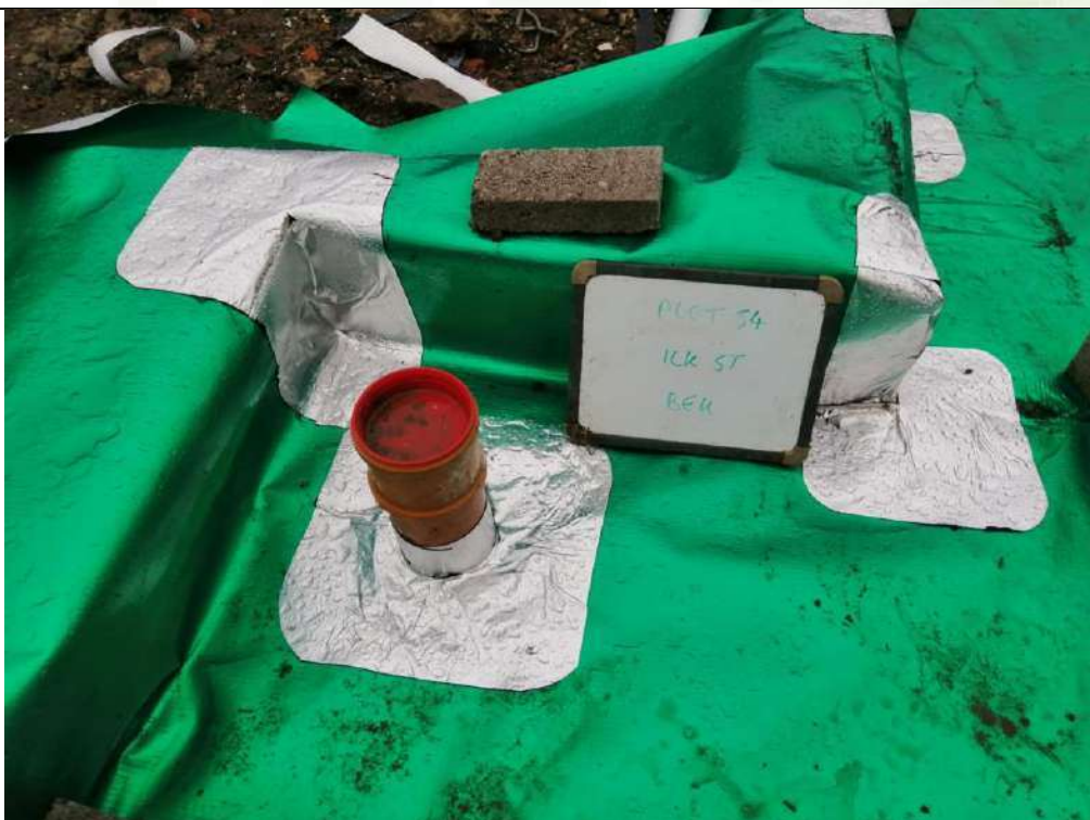
Photograph 6: Validation of Gas Membrane Installation
