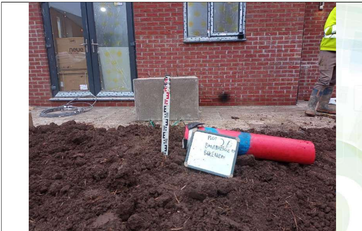
Photograph 2: Validation of Garden Capping Thickness
