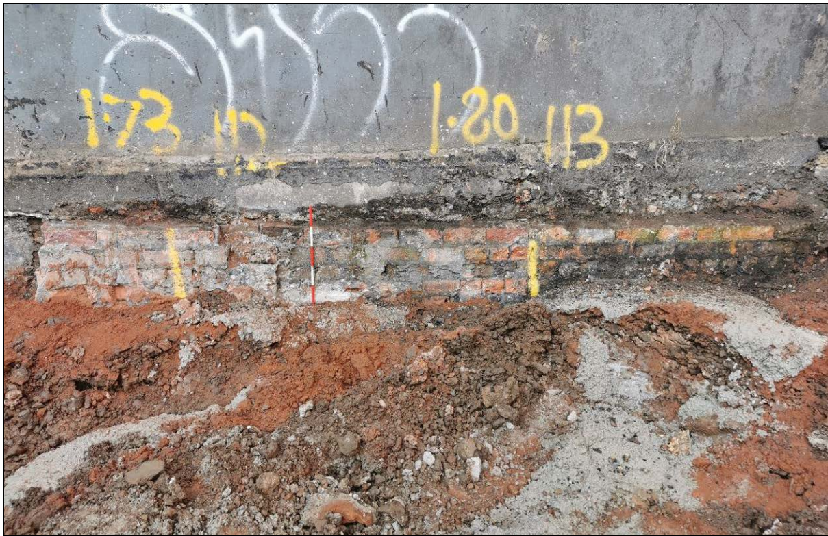
Plate 5: Side wall, looking towards Abingdon Street, towards the rear of the property
