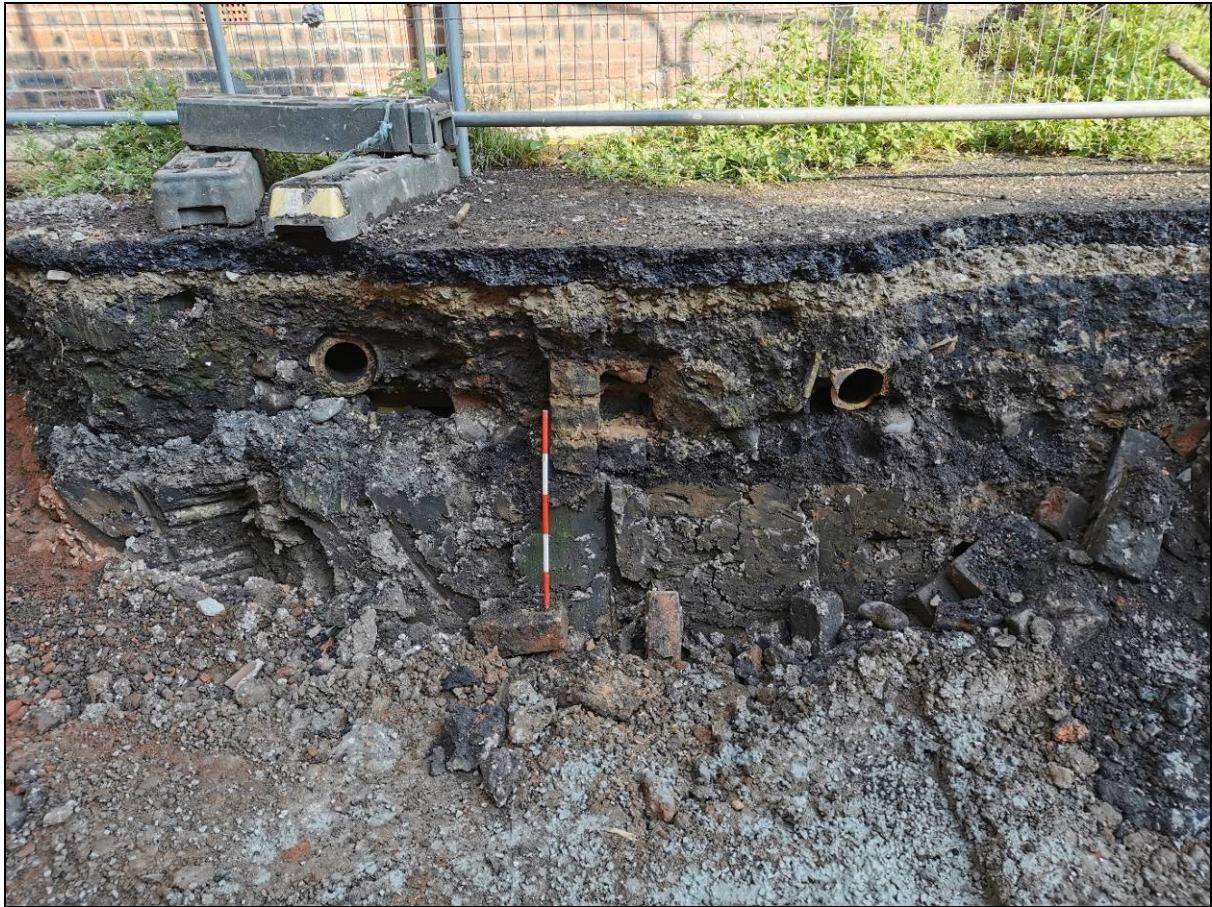
Plate 8: Drains at rear of property, looking towards Bloom Street.
