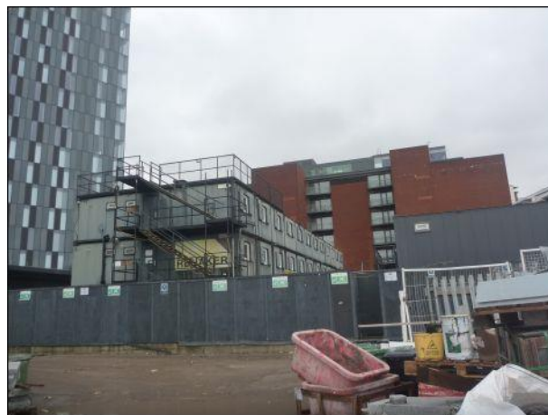
Photo 12: Building 2, south-western and south-eastern elevations
