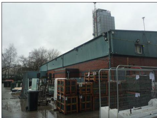
Photo 9: Building 1, south-western elevation
