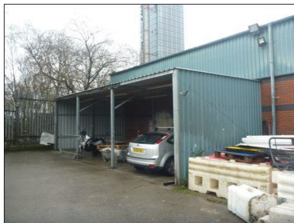
Photo 10: Single-storey extension at Building 1
