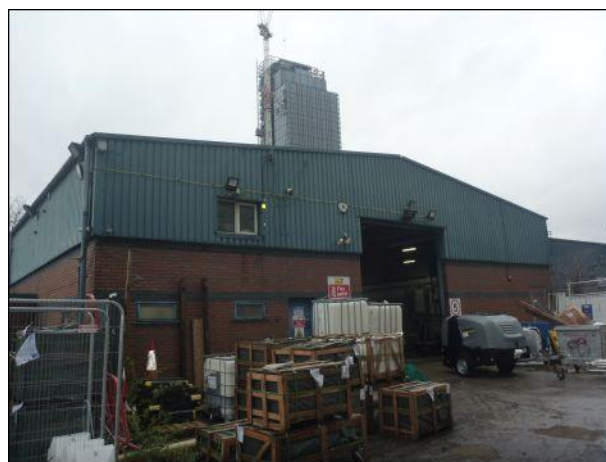
Photo 8: Building 1, south-eastern elevation
