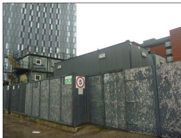
Photo 14: Metal storage containers
