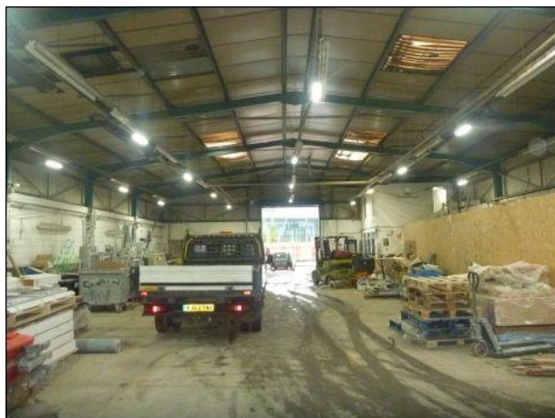
Photo 11: Building 1, internal area
