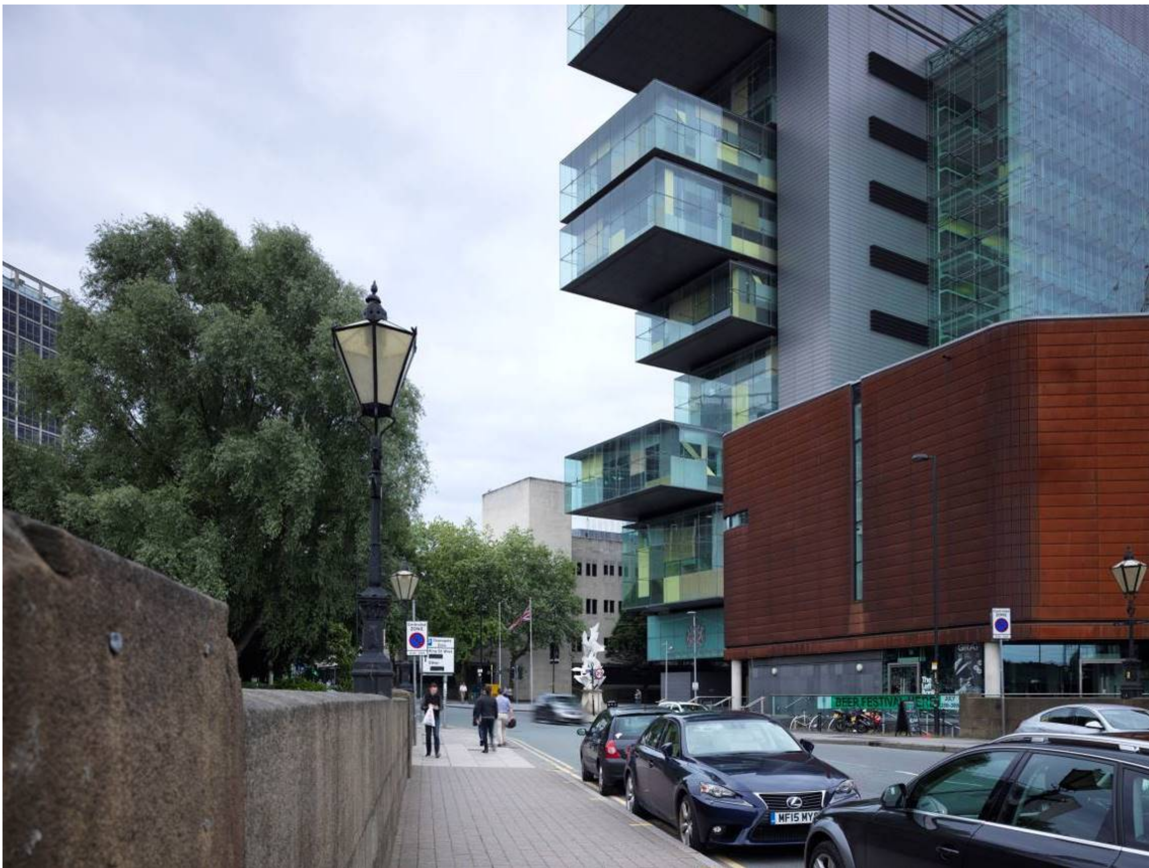
Figure 19A: View 16, above. As existing.
