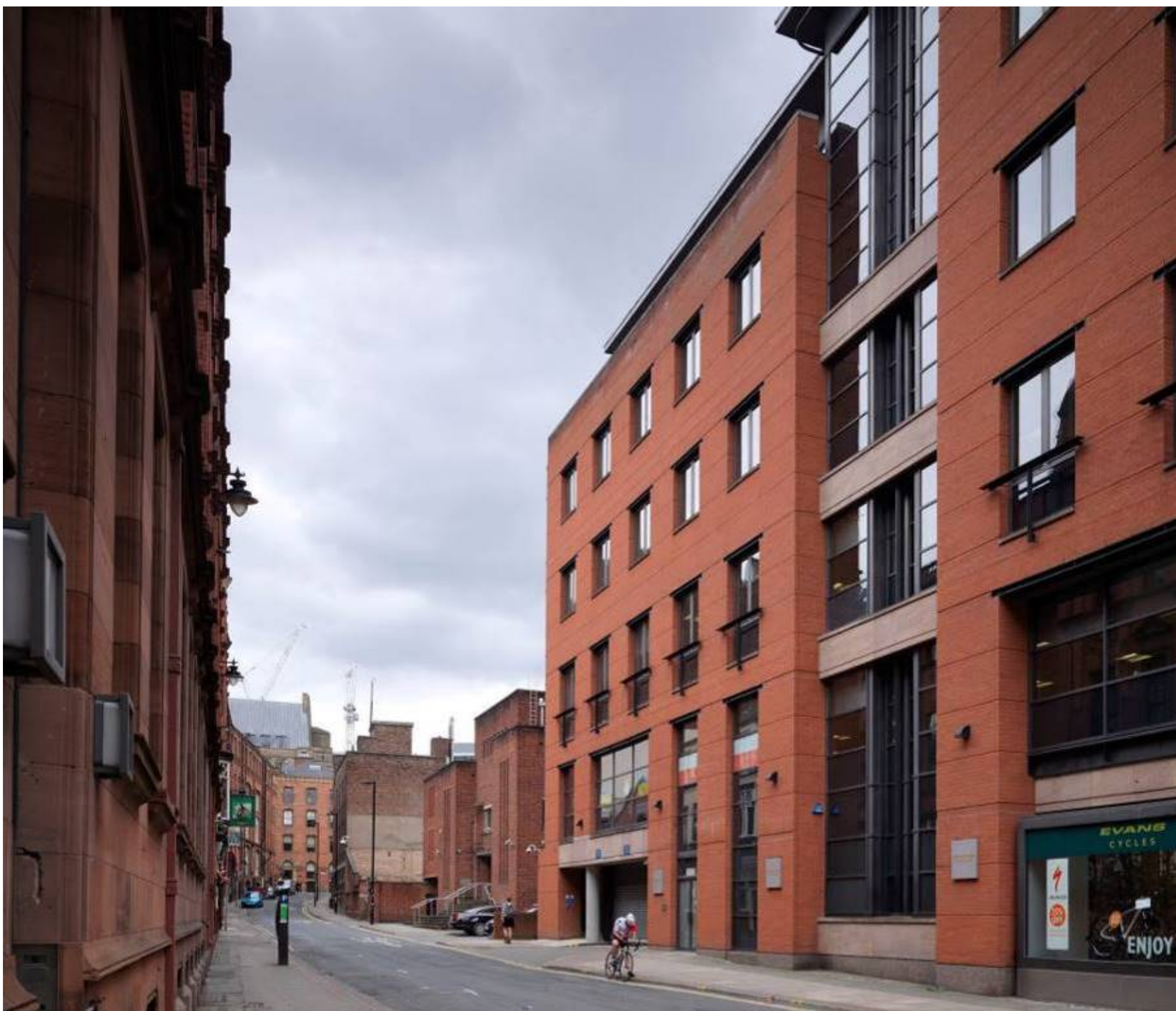
Figure 5A: View 2, above. As existing.
