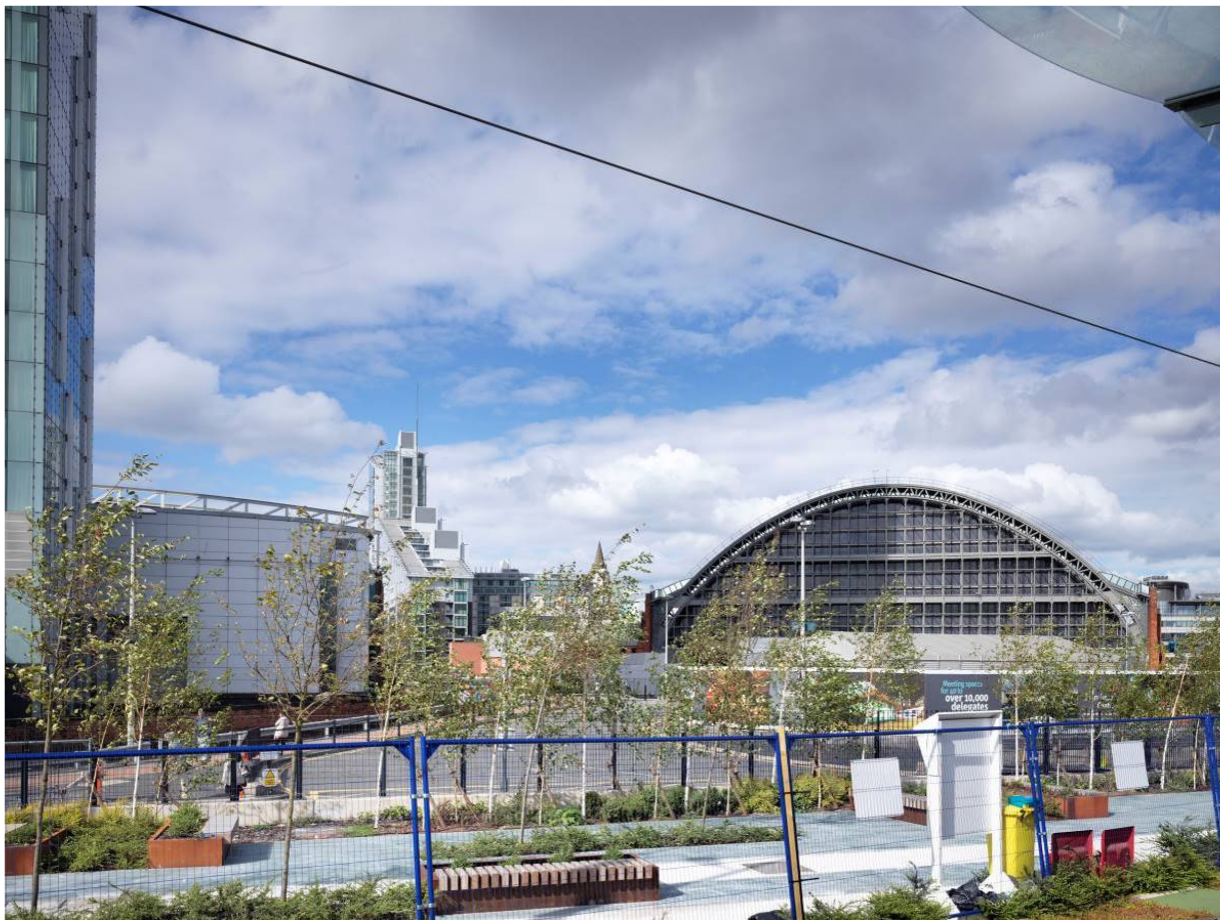
Figure 11A: View 8, above. As existing.
