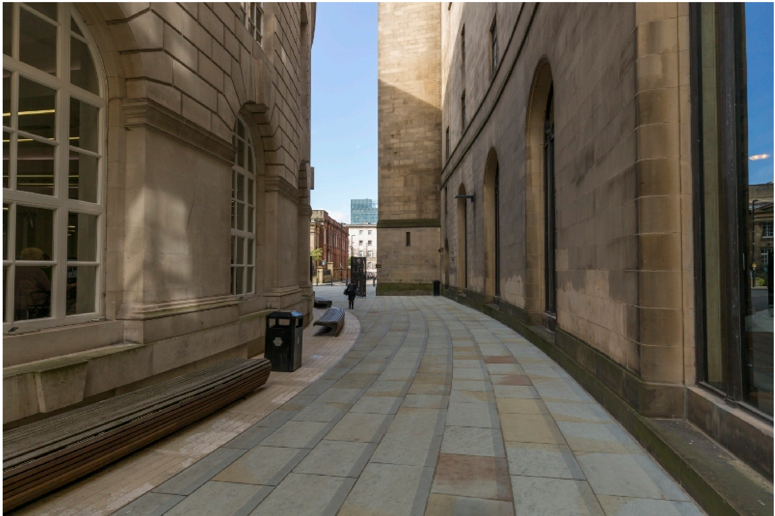
Figure 9A: View 6, above. As existing.
