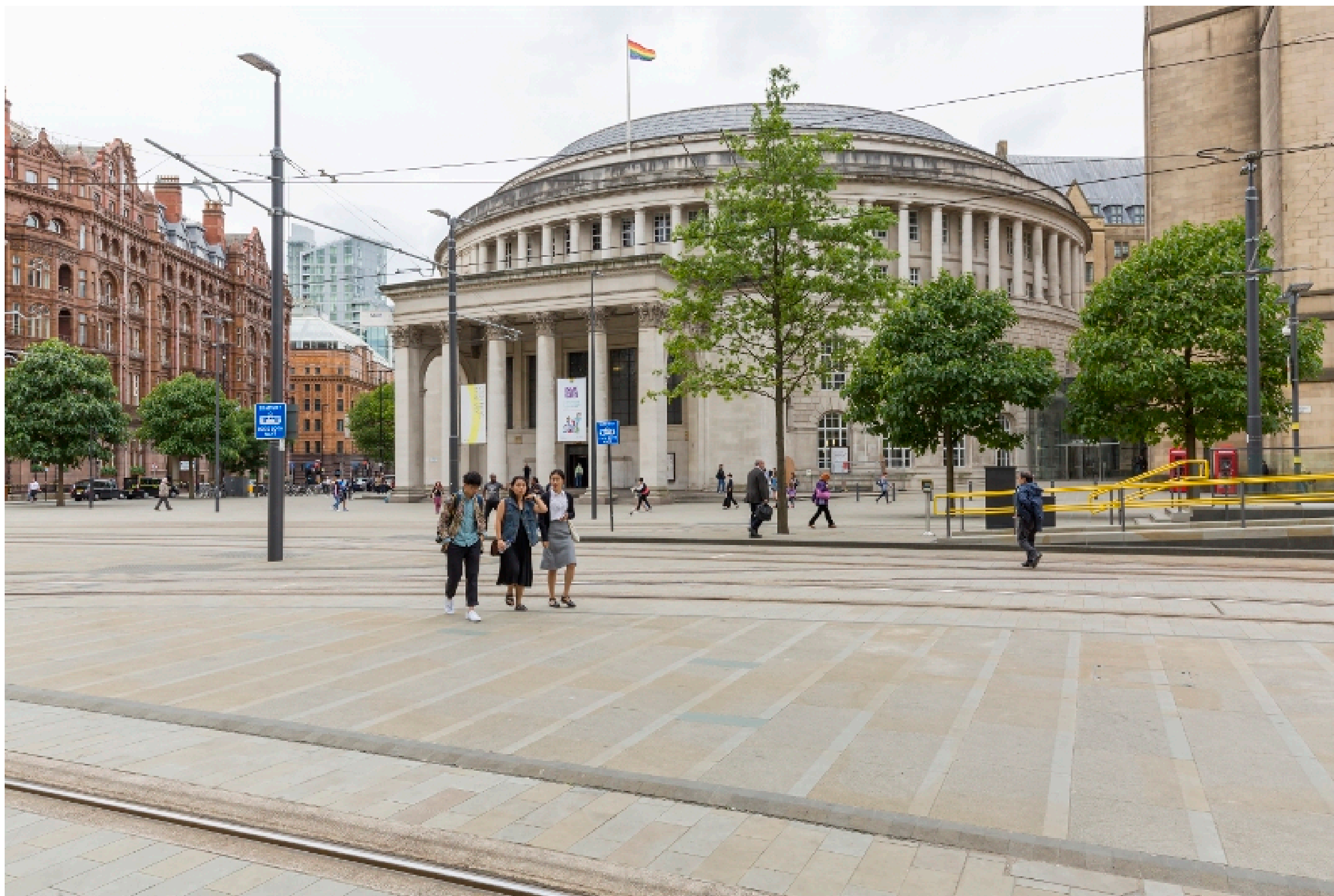
Figure 10A: View 7, above. As existing.
