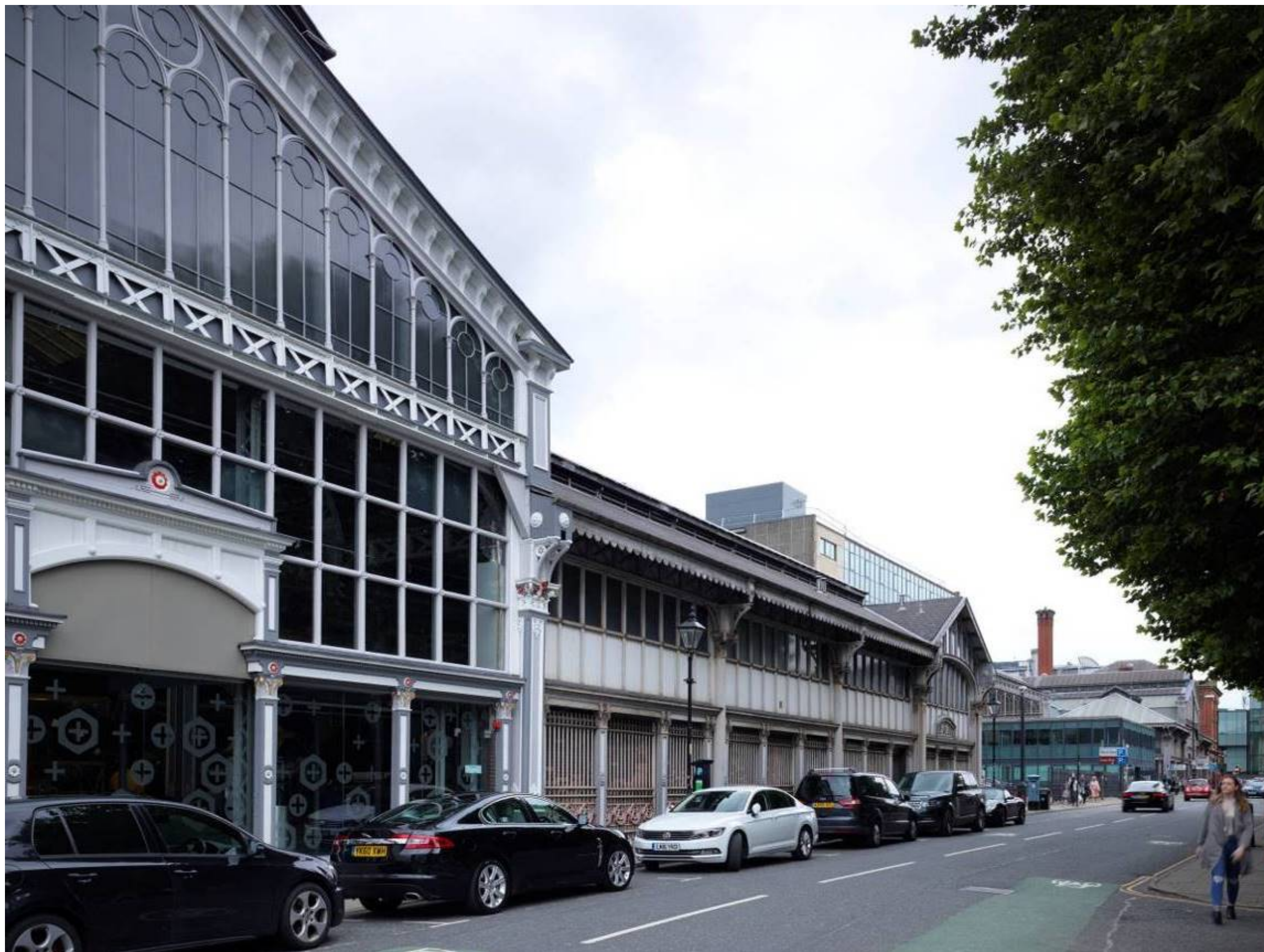
Figure 18A: View 15, above. As existing.
