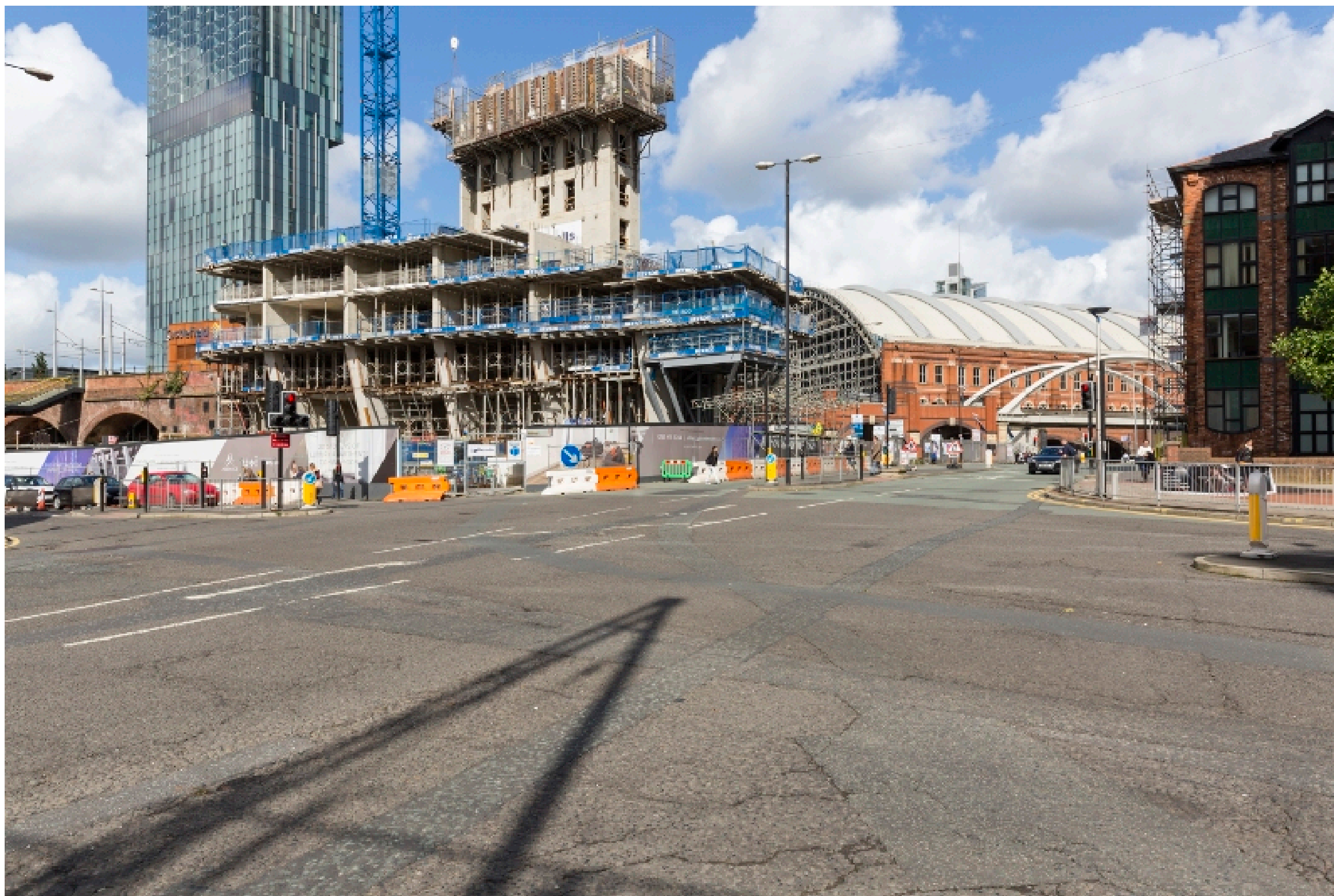
Figure 15A: View 12, above. As existing.
