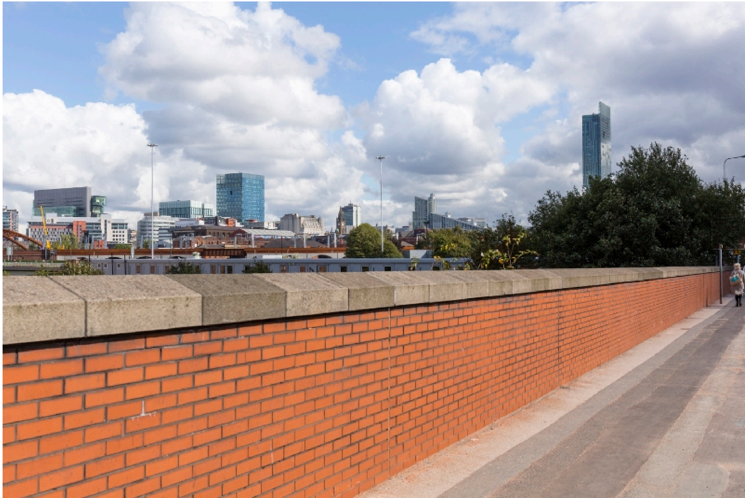
Figure 17A: View 14, above. As existing.
