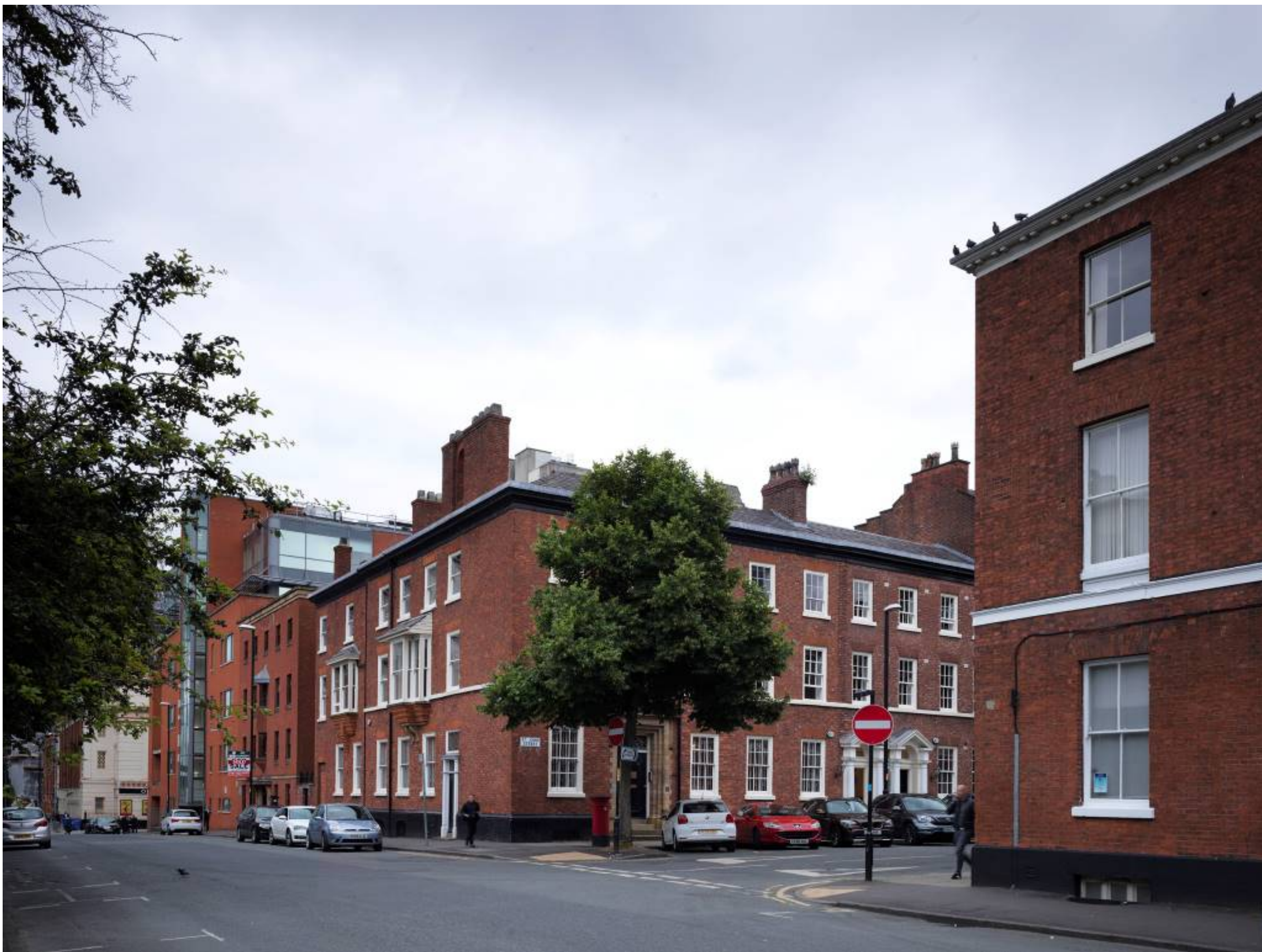
Figure 14A: View 11, above. As existing.
