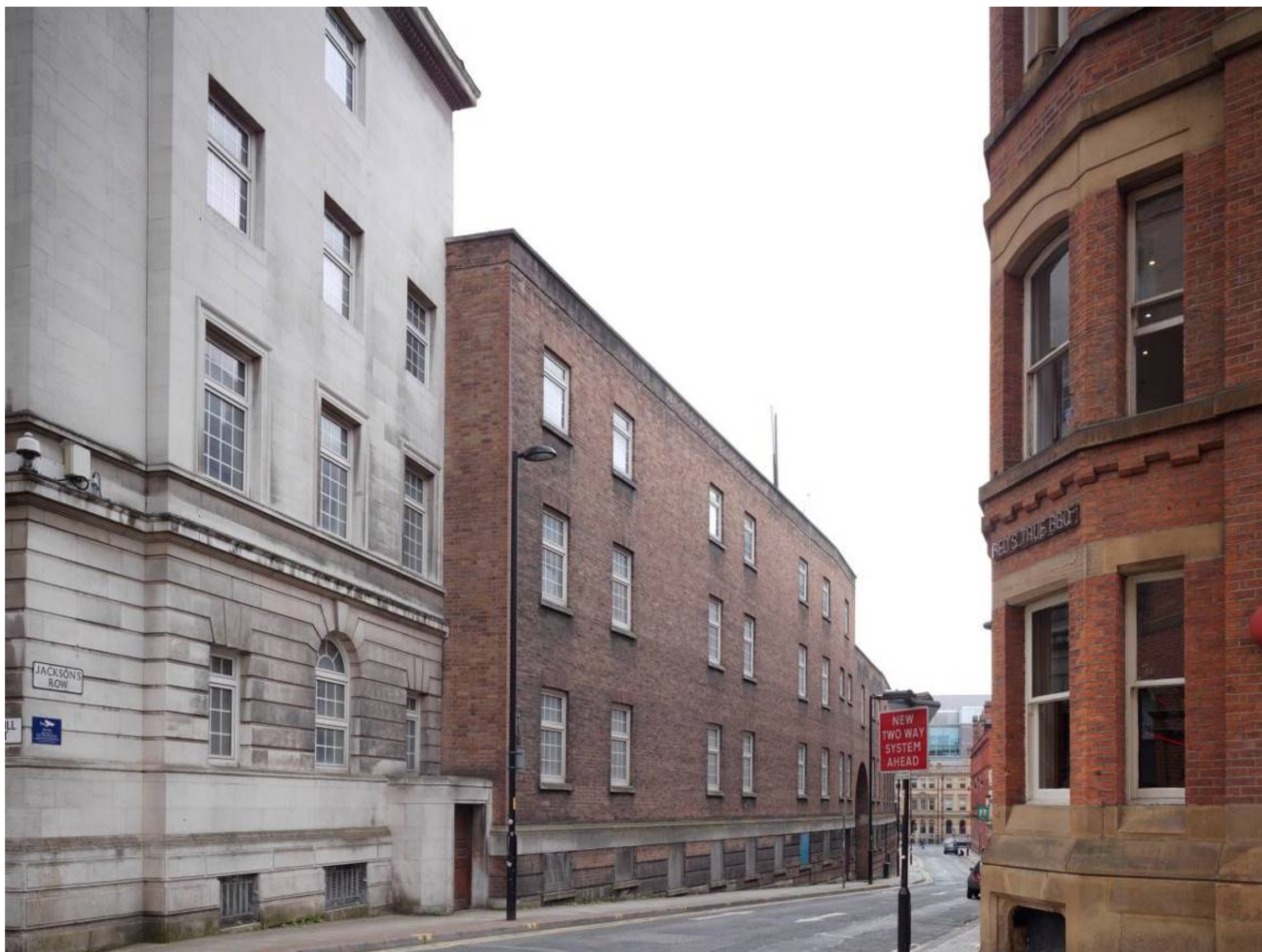
Figure 4A: View 1, above. As existing.
