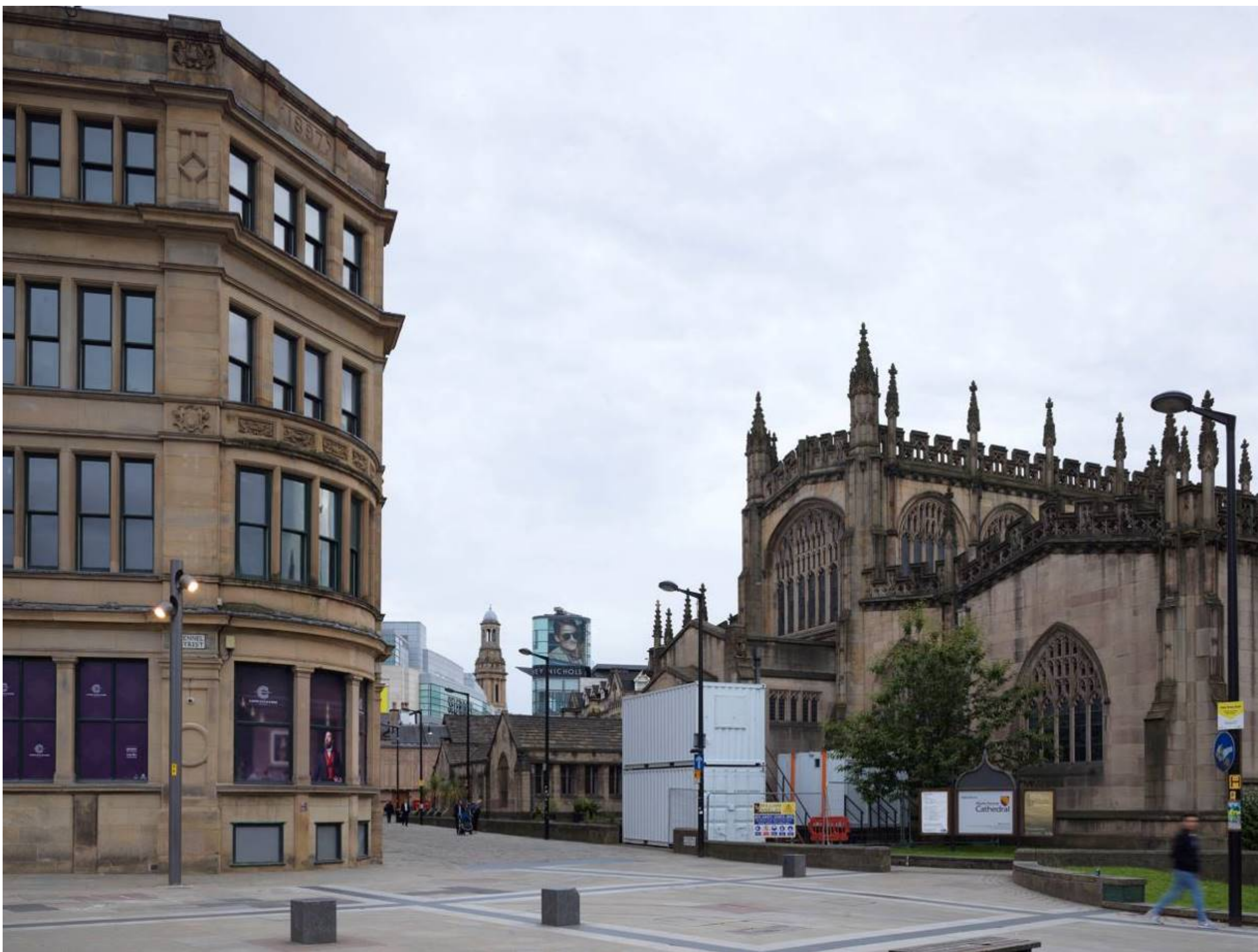
Figure 20A: View 17, above. As existing.
