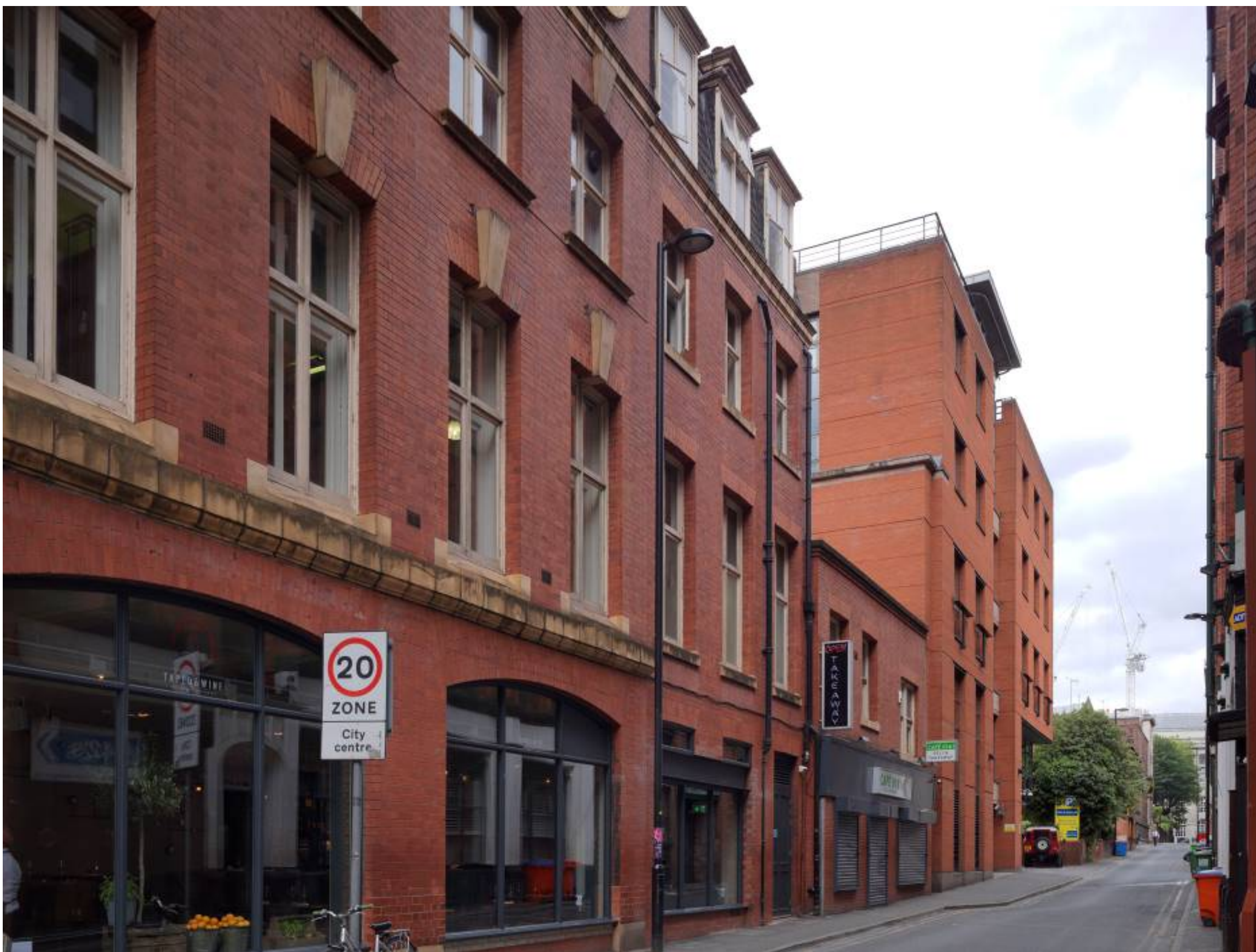
Figure 7A: View 4, above. As existing.
