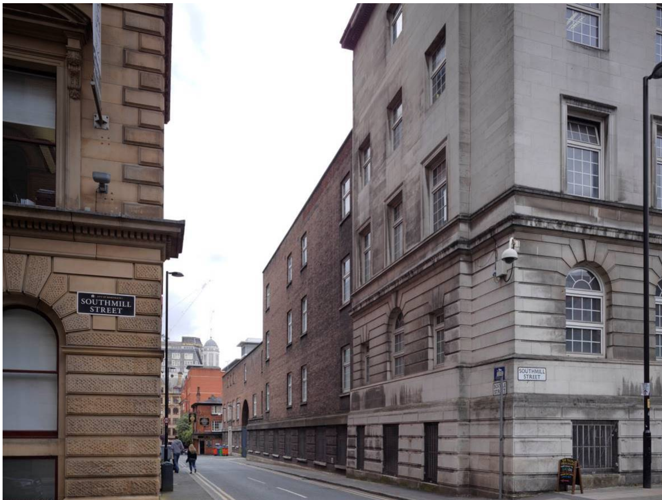
Figure 6A: View 3, above. As existing.
