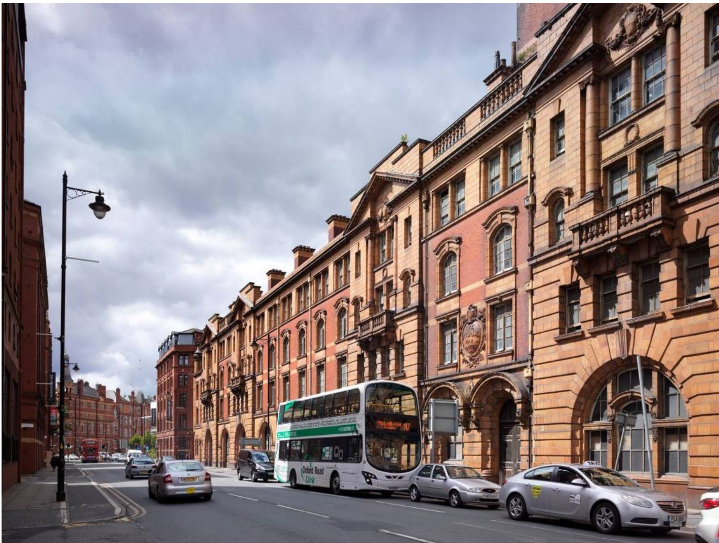
Figure 24A: View 21, above. As existing.
