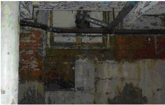
PRINCESS STREET BASEMENT UNIT 4 WINDOWS
