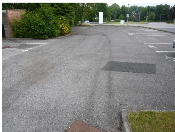
Photo 2: Area of car park within site, facing north
