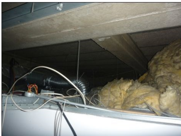
Photo 13: Building 1, void above former supermarket
