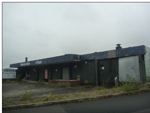
Photo 6: Building 1, south-eastern elevation
