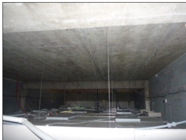
Photo 14: Building 1, void above former supermarket
