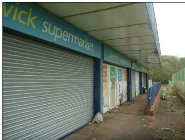
Photo 8: Building 1, south-western elevation, northern end
