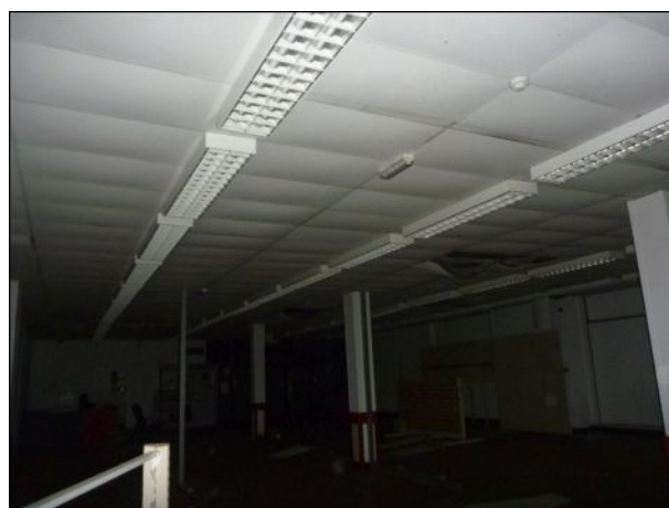
Photo 12: Building 1, former supermarket
