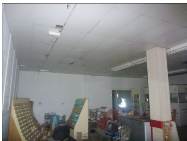
Photo 11: Building 1, former supermarket
