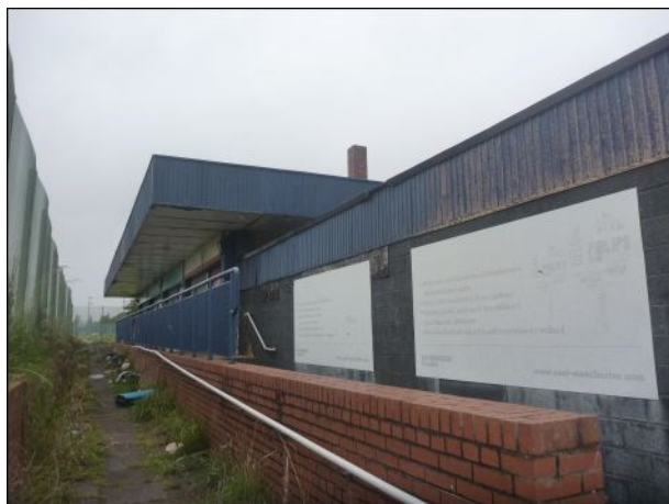
Photo 7: Building 1, south-western elevation, southern end
