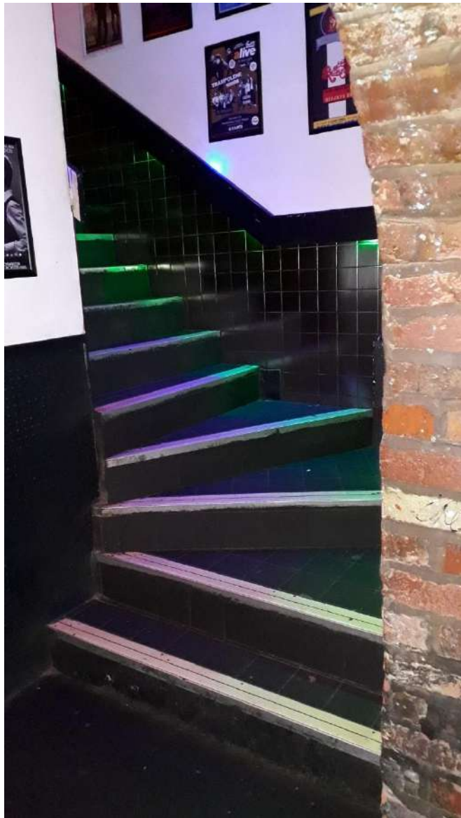
Current entrance to lower ground nightclub from Princess Street elevation. This staircase to be replaced with a compliant staircase for escape purposes only
