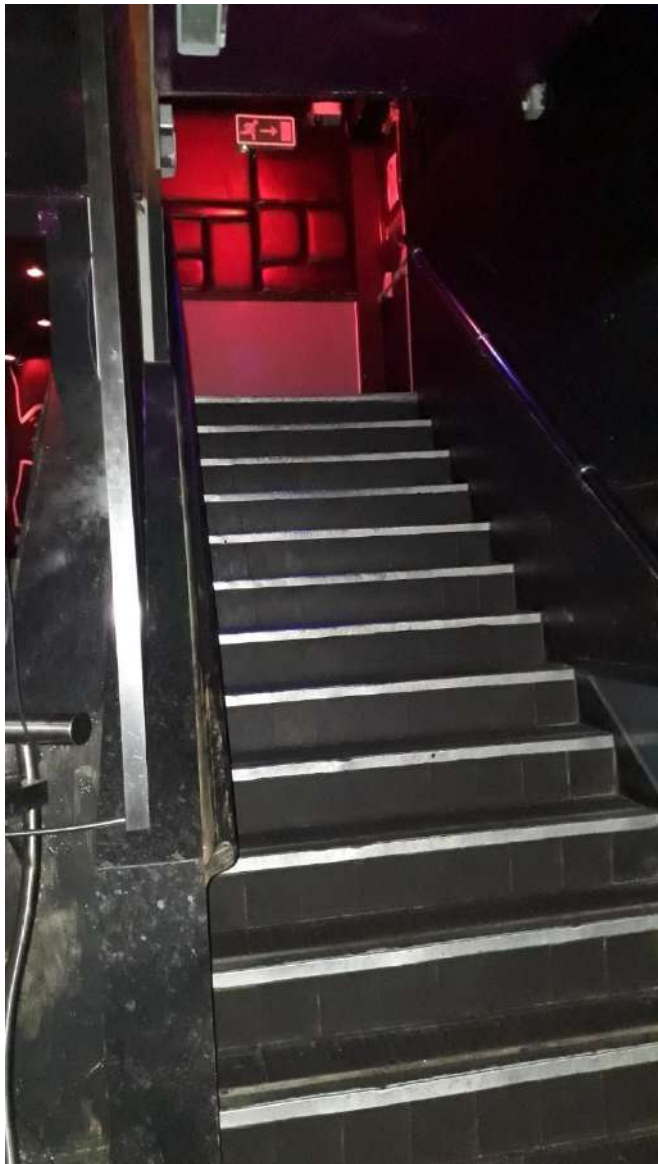
Current Fire Escape stairs from lower ground nightclub out to Bloom Street. These will become the new point of entry to the Lower Ground floor nightclub going forward
