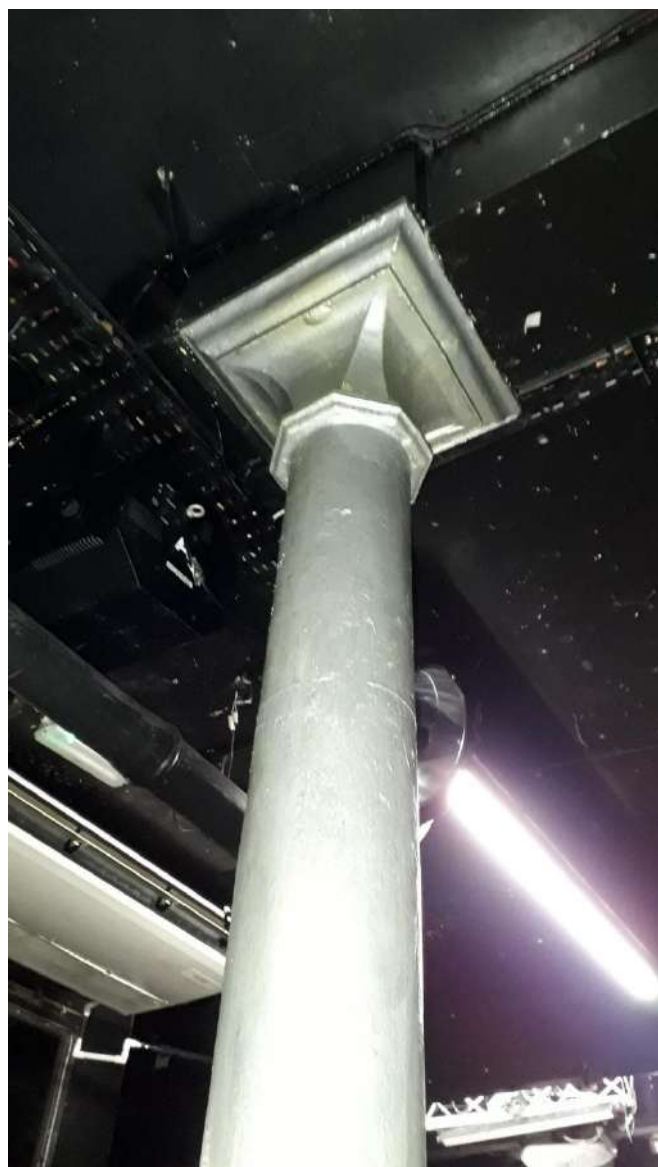
Existing cast iron columns to nightclub floors
