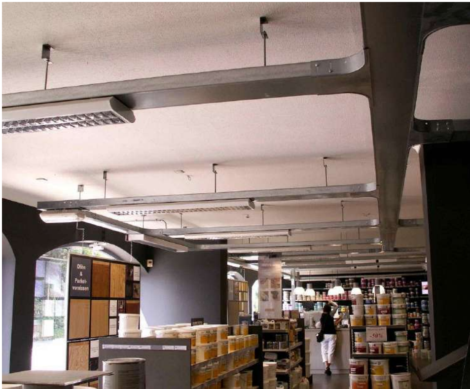
Industrial trunking for power and lighting distribution, exposed cable trays and ductwork, bench office furniture, exposed joists in certain areas.
