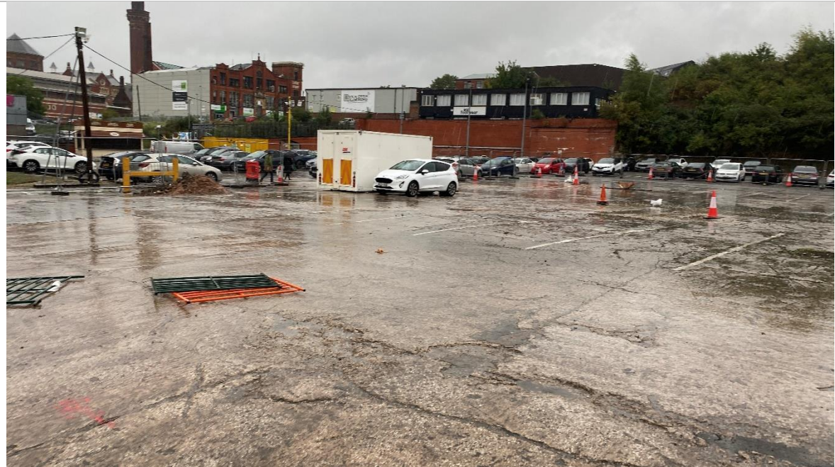
PLATE 2 VIEW OF SITE FACING NORTHEAST TOWARDS THE RETAINING WALL (OFF-SITE)
