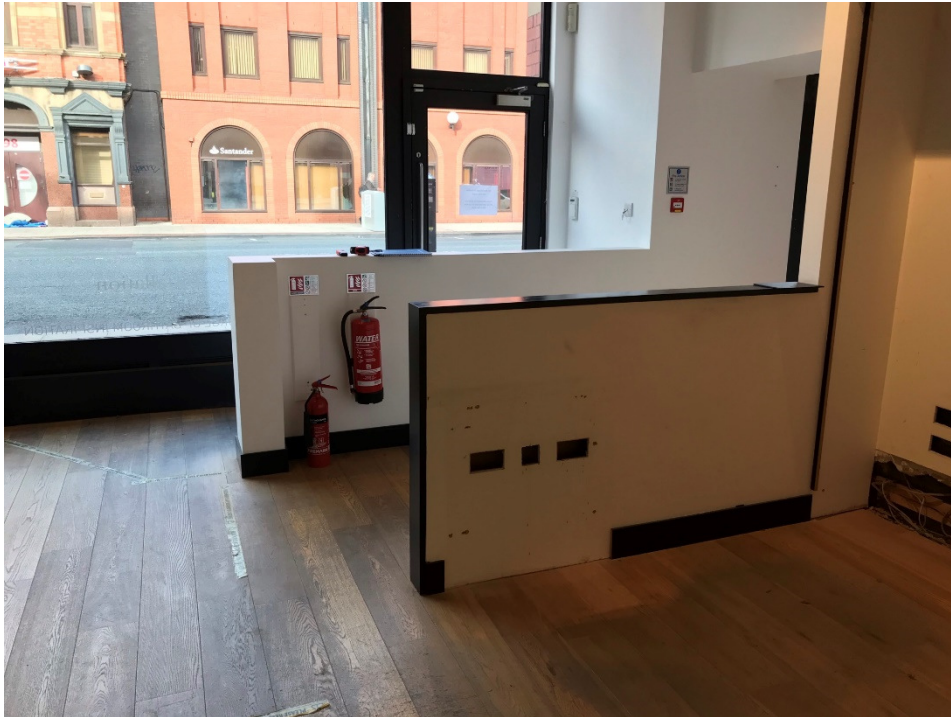
1. Internal view of main access door to Unit 267.
