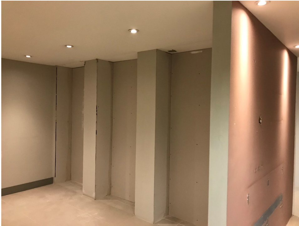
11. General view of staircase to Unit 263.
