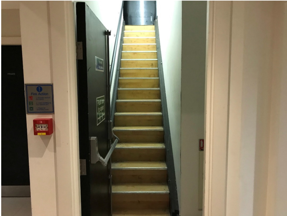
9. General view of staircase to Unit 265, this stairs will solely serve proposed Units 265/267.
