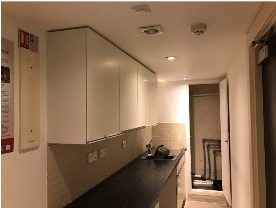
16. General view of existing kitchen to Unit 261, to be retained.
