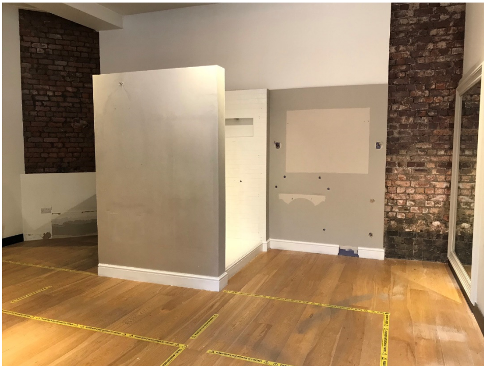
2. General view of existing condition of Unit 265.
