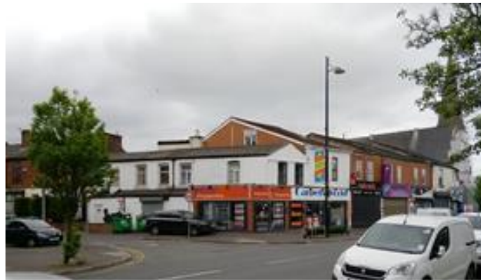
Fig. 2 - Application site at the junction of Stockport Road and Balleratt Street
