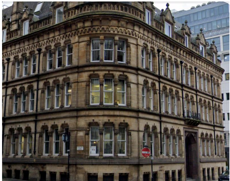
Figure 5 – View of the existing façade which is to be retained.
