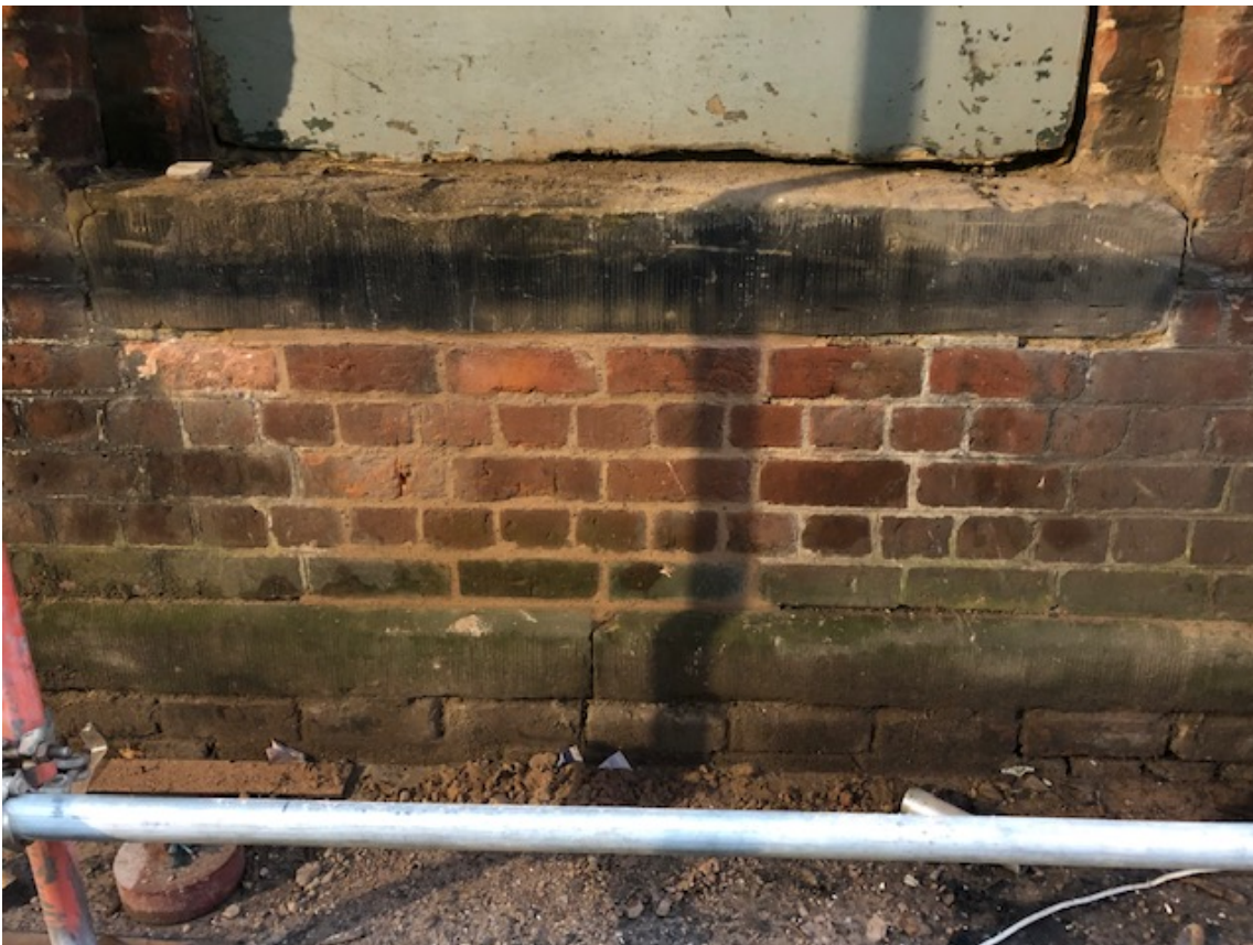
fig01: cleaning sample undertaken to minshull house @ ground floor
